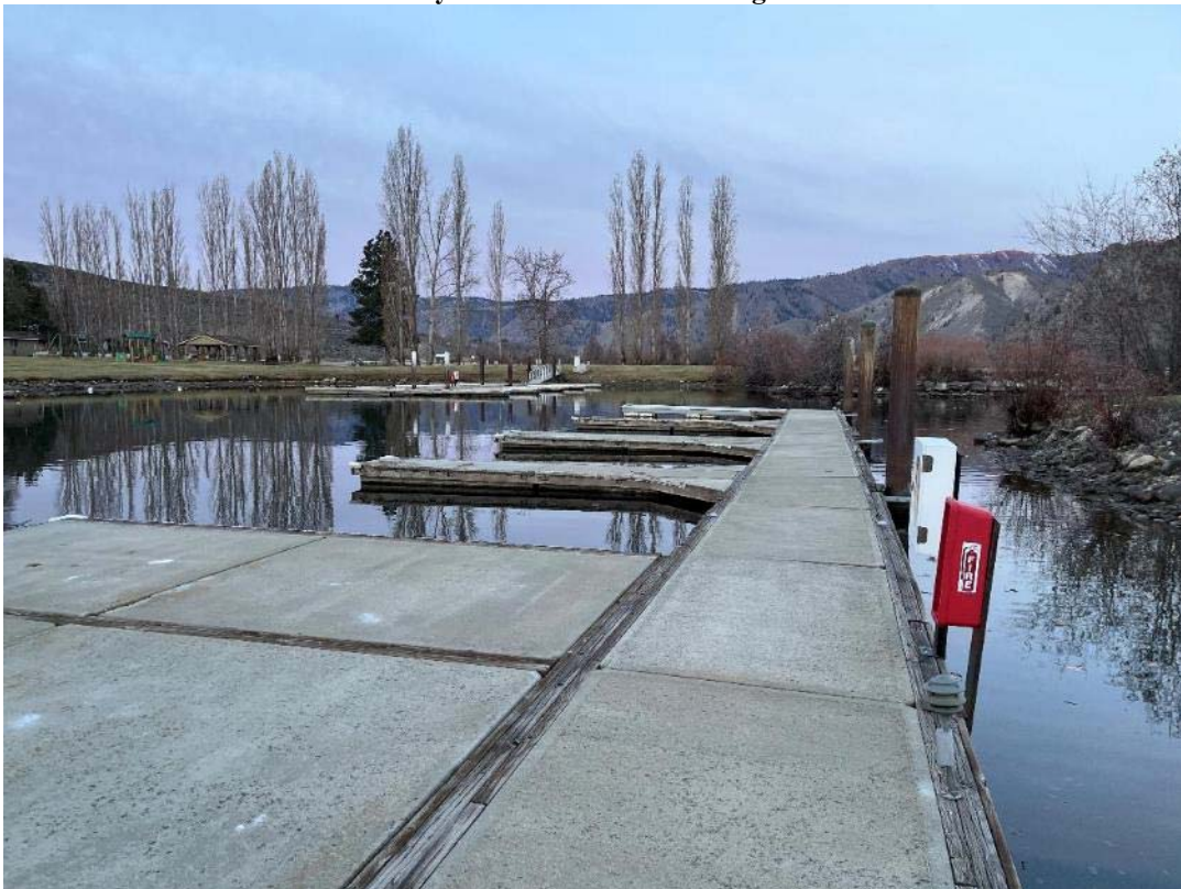
Photograph 7. Existing concrete float (larger float) in the middle basin to be removed and replaced with a fully grated float system that will be reconfigured.
