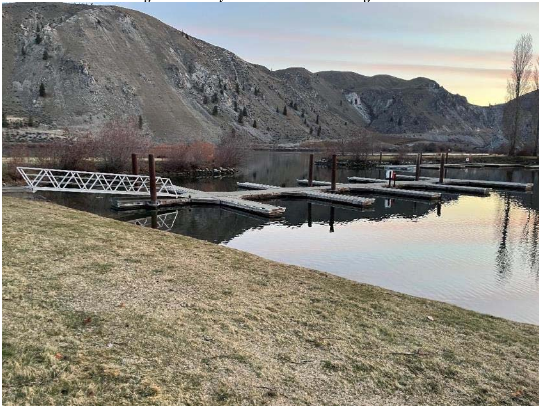
Photograph 9. Existing concrete float (smaller float) in the middle basin to be removed and replaced with a fully grated float system that will be reconfigured.
