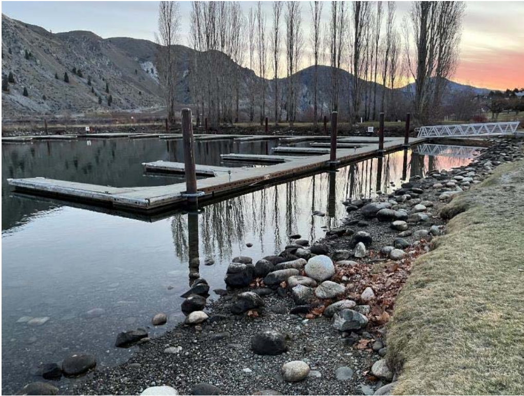
Photograph 4. Existing concrete float (larger float) in the middle basin to be removed and replaced with a fully grated float system that will be reconfigured.
