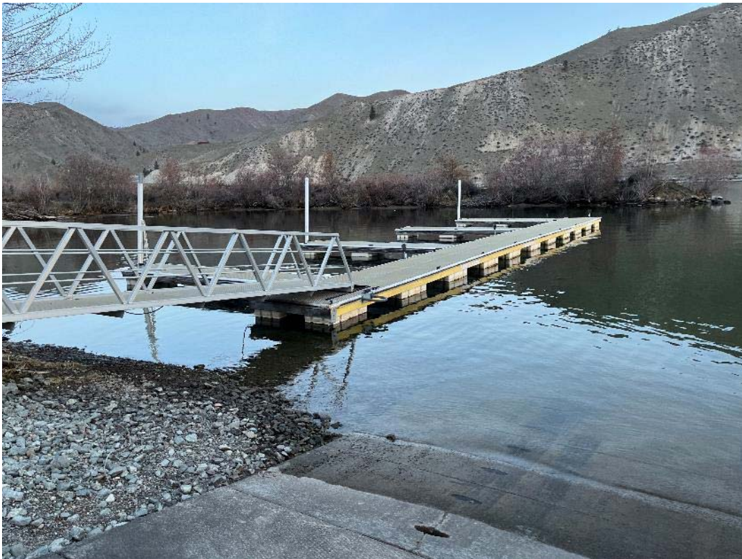
Photograph 15. Existing wooden float in the downriver basin (downriver float) to be removed and replaced a floats slightly larger floats (additional slip at waterward end).
