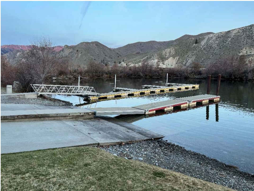
Photograph 13. Existing wooden launch handling float in the downriver basin to be removed and replaced with same sized float.
