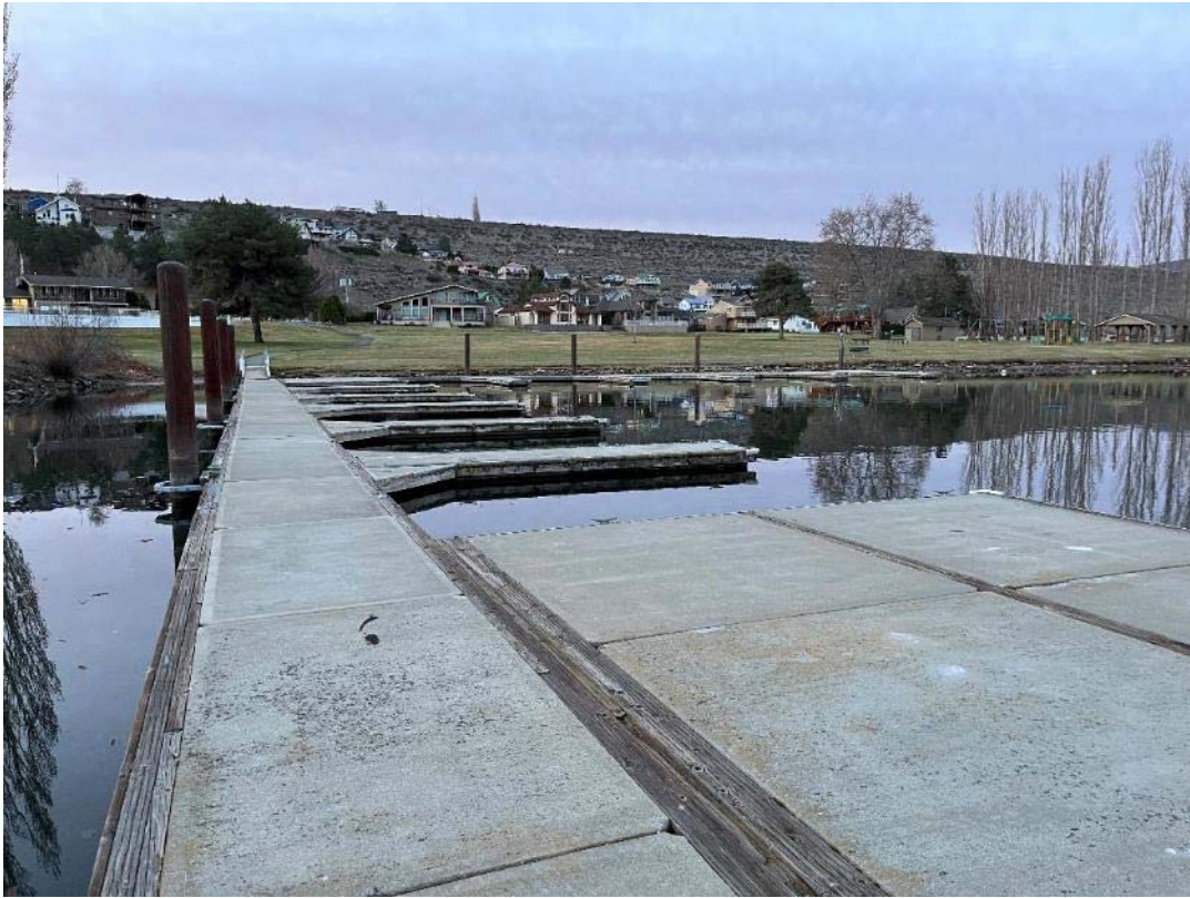
Photograph 6. Existing concrete float (larger float) in the middle basin to be removed and replaced with a fully grated float system that will be reconfigured.
