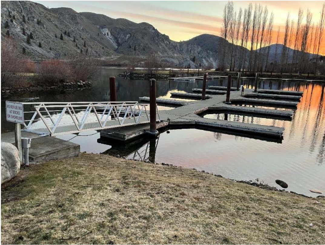
Photograph 8. Existing concrete float (smaller float) in the middle basin to be removed and replaced with a fully grated float system that will be reconfigured.
