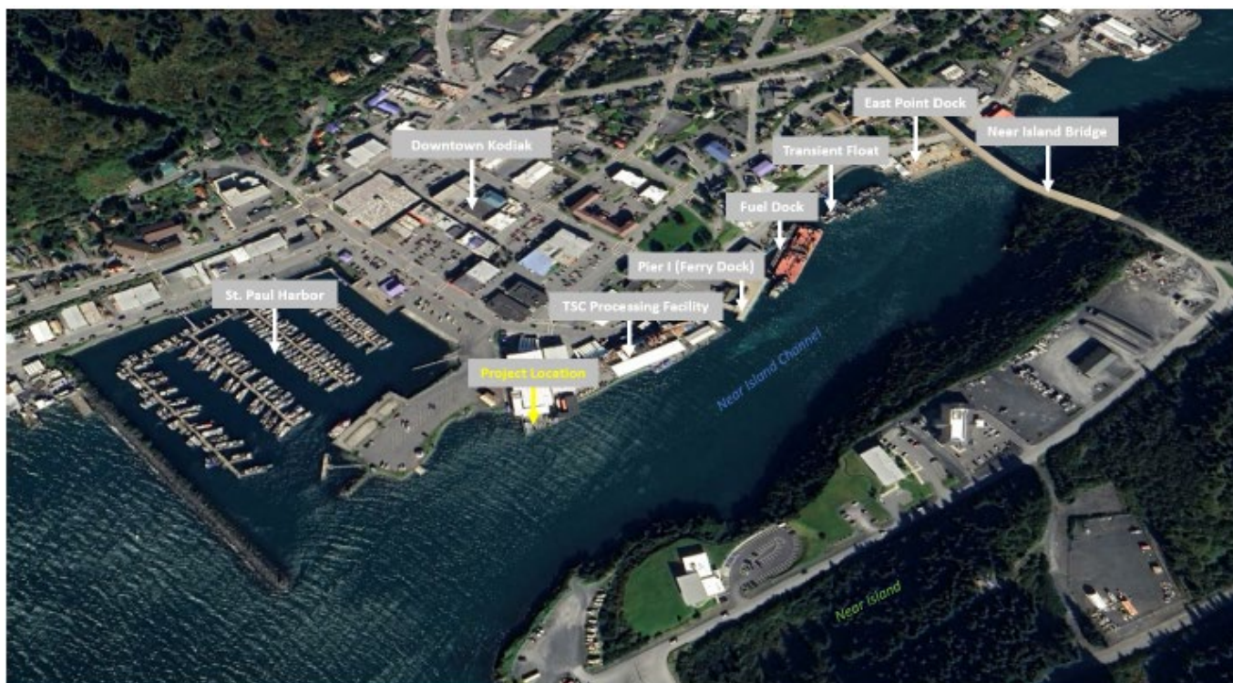
Figure 1. Location of the Trident bunkhouse dock to be replaced (in yellow text) and other relevant landmarks.
