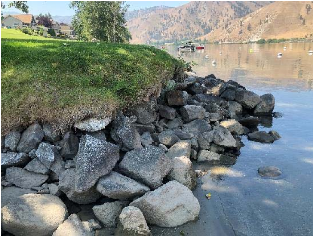
Photograph 13. Existing armored shoreline immediately downriver of the launch that will be removed to eliminate sedimentation at the launch.
