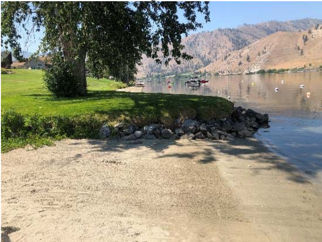
Photograph 12. Existing vegetation and armored shoreline conditions immediately downriver of the launch that will be removed to eliminate sedimentation at the launch.
