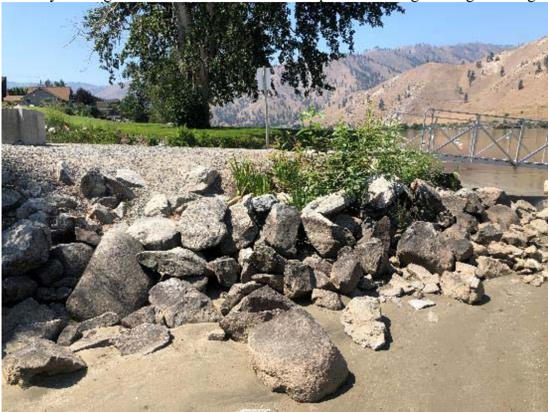
Photograph 10. Existing vegetation and shoreline conditions immediately upriver of the launch to be removed. Shoreline will be restored and protected using gravel/cobble, soil bags, and vegetation.
