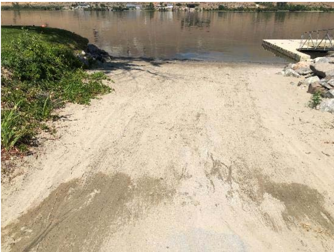
Photograph 4. Existing boat launch at Bauers Landing Community Shoreline covered with naturally deposited sand; to be removed.
