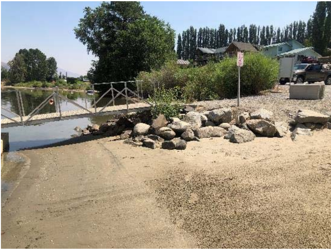
Photograph 3. Existing launch handling float at the Bauers Landing launch and concrete abutment and armored shoreline to be removed.
