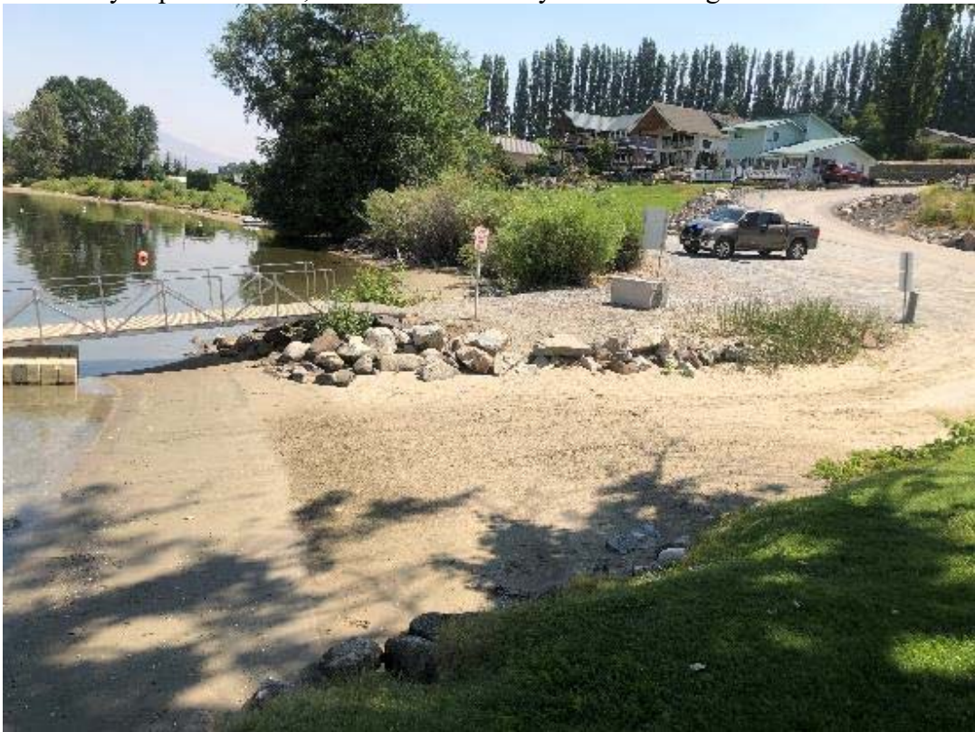
Photograph 6. Existing boat launch at Bauers Landing Community Shoreline covered with naturally deposited sand; to be removed. Jetty with handling float to be removed.
