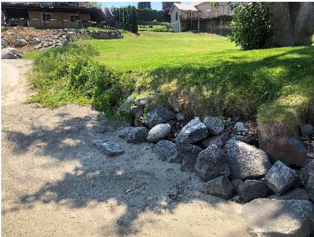
Photograph 14. Existing armored shoreline immediately downriver of the launch that will be removed to eliminate sedimentation at the launch.
