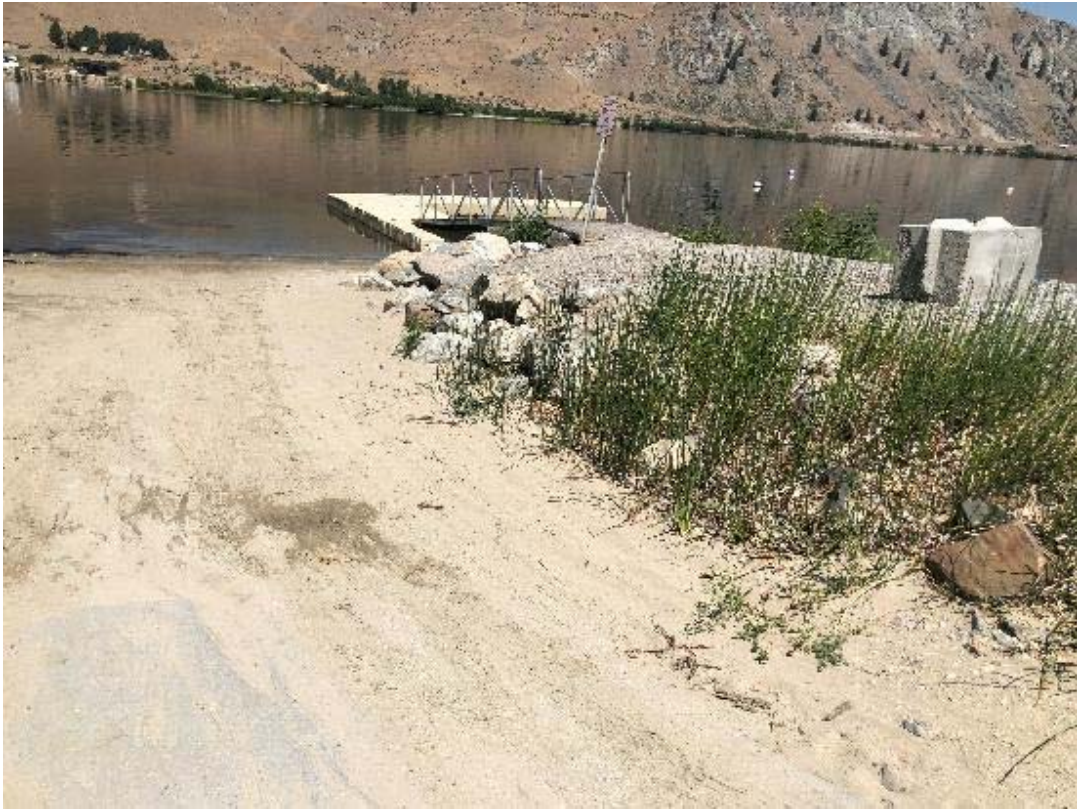
Photograph 5. Existing boat launch at Bauers Landing Community Shoreline covered with naturally deposited sand; to be removed. Jetty with handling float to be removed.
