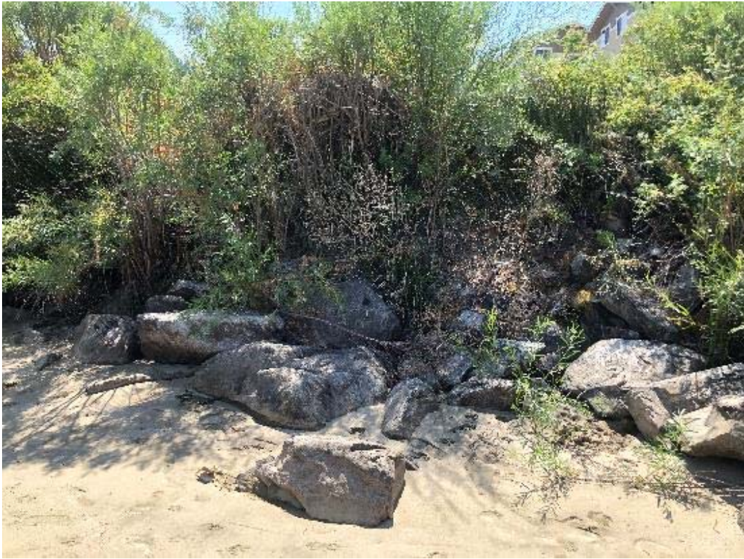
Photograph 9. Existing vegetation and shoreline conditions immediately upriver of the launch that is currently eroding. Shoreline will be restored and protected using soil bags and vegetation.
