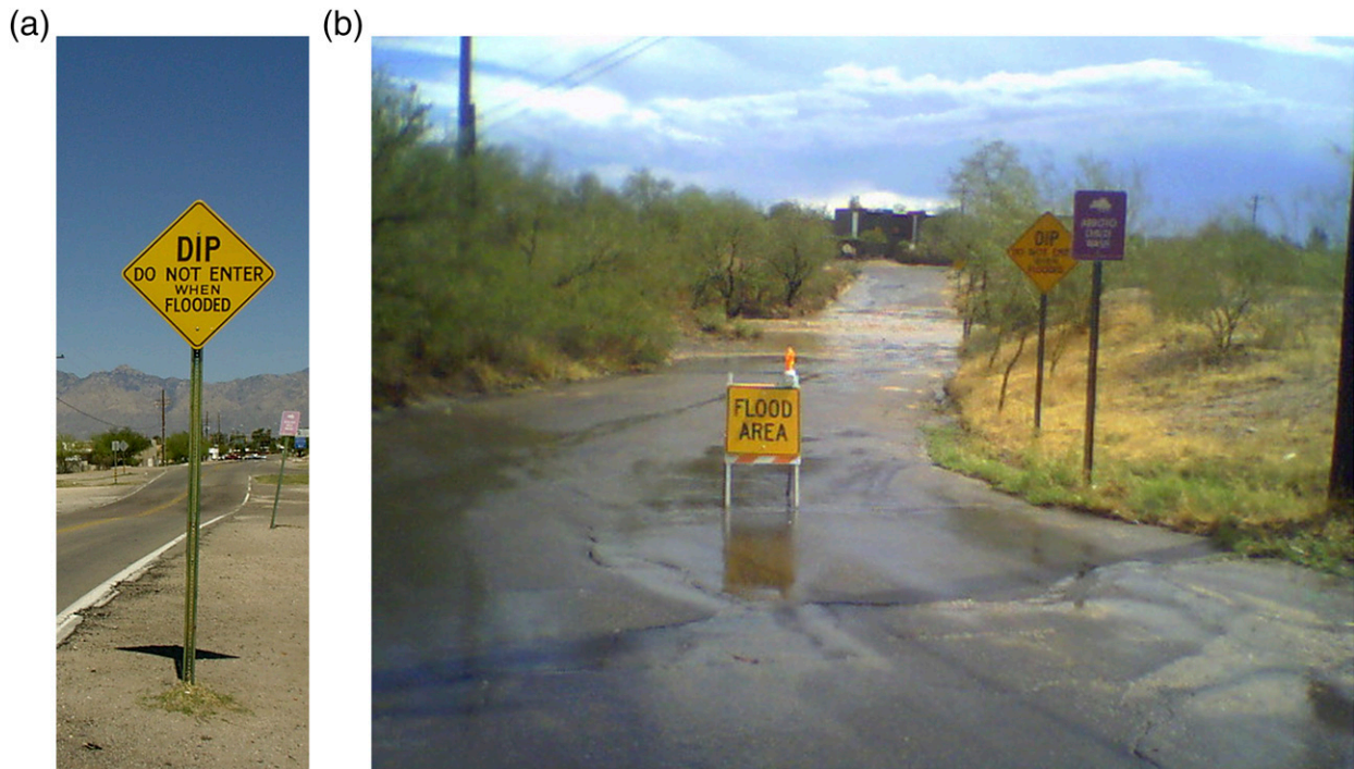
FIG. 1. Types of flood signs: (a) dip sign at Sarnoff Road and 24th Street and (b) dip sign and A-frame on Highland Avenue at the Arroyo Chico Wash while flooded to a depth of \sim 4 ft (1.2 m). This particular dip crossing was recently eliminated by the installation of a bridge and culvert. Photograph credits: A. Coles.
