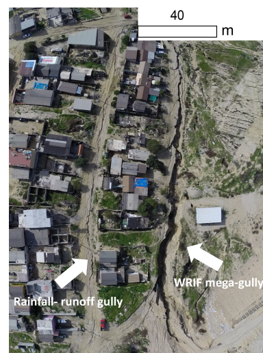
Figure 7. High-resolution photograph showing the contrast between gullies generated by rainfall–runoff only (road on left) and mega-gully B (road on right).
