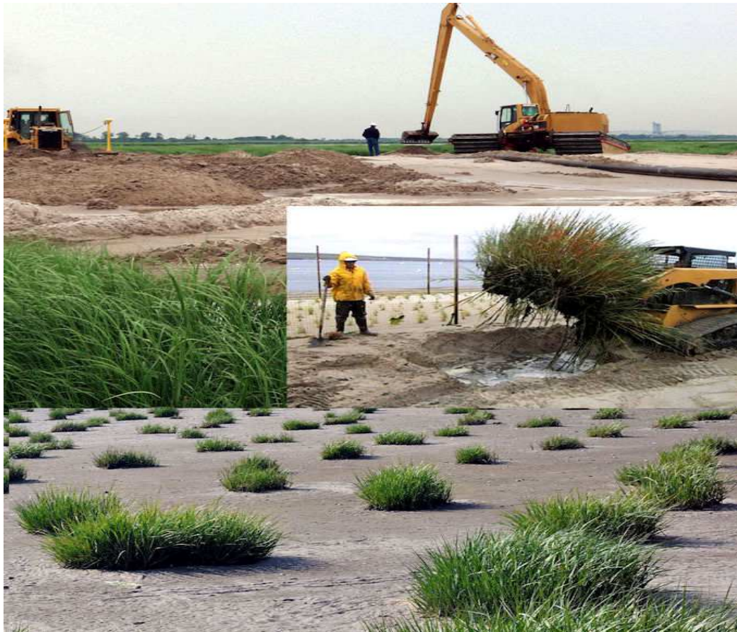
Figure 7. Replanting of salt marsh grass, Jamaica Bay, New York. (Source: United States Army Corps of Engineers).
