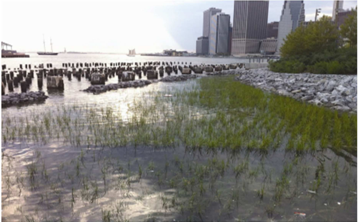
Figure 8. Soft edge “living shoreline”, Brooklyn Bridge Park, New York City. (Source: New York City Department of City Planning, 2013).
