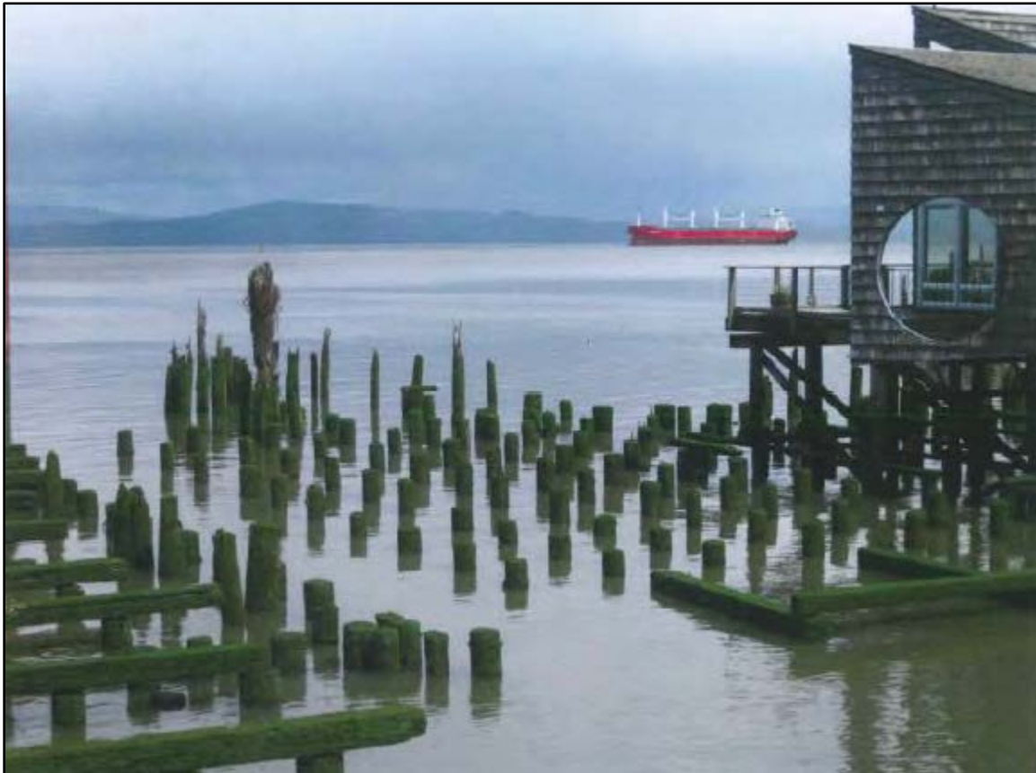
Figure 6. Waterward view of existing conditions at the construction site.
