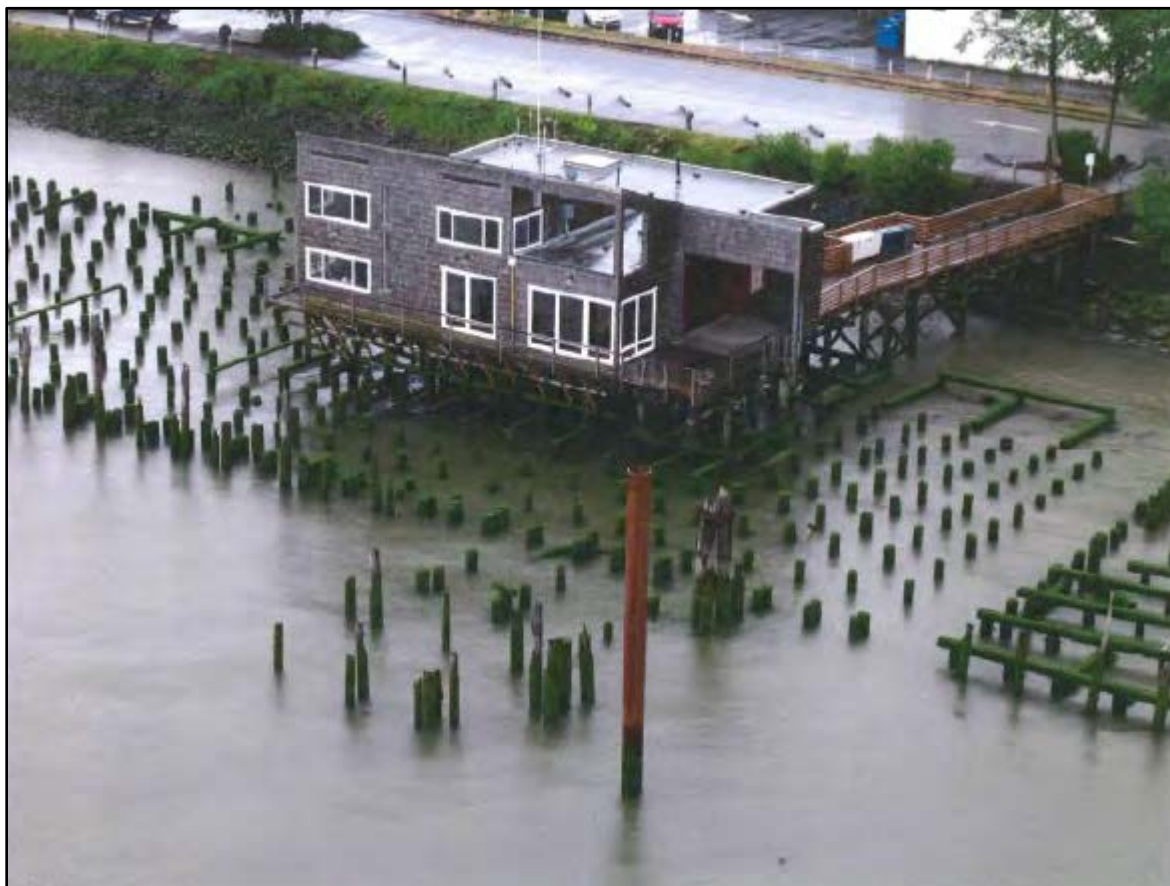
Figure 5. Baseline conditions at the proposed construction site.
