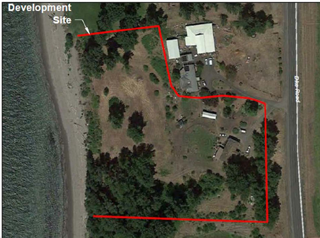
Figure 10. Baseline conditions at the proposed marine terminal construction site.
