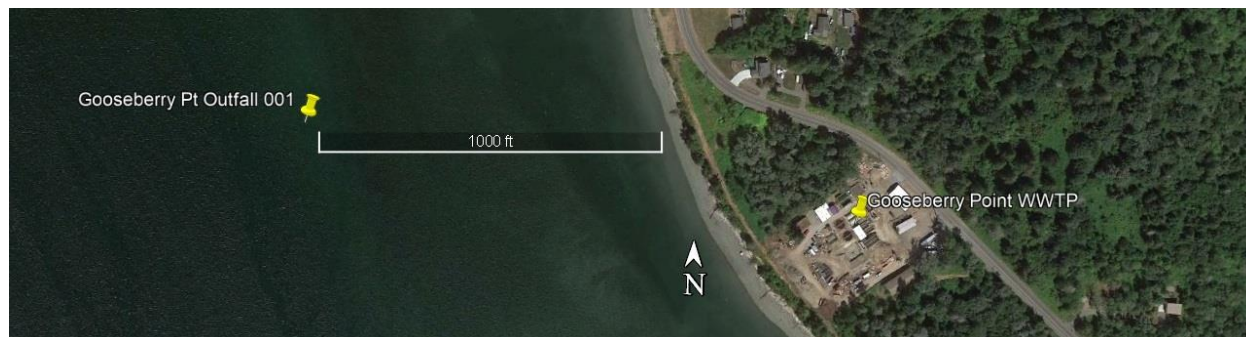
Figure 2. Google Earth photograph showing the Lummi Gooseberry Point WWTP and the approximate location of its outfall.
