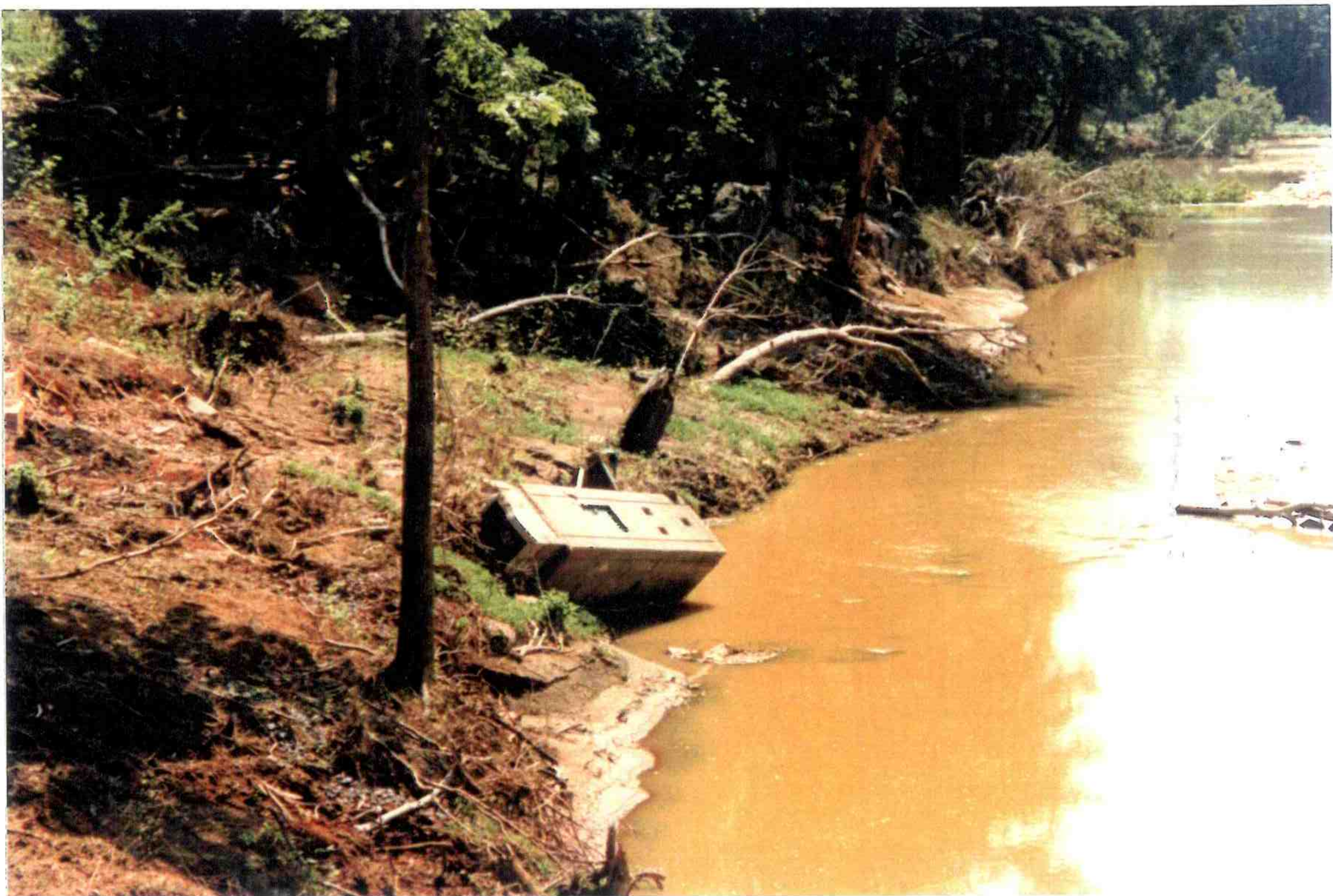
Picture 2: USGS streamgage on Rapidan River in Greene County after flood waters washed it off its foundation.
