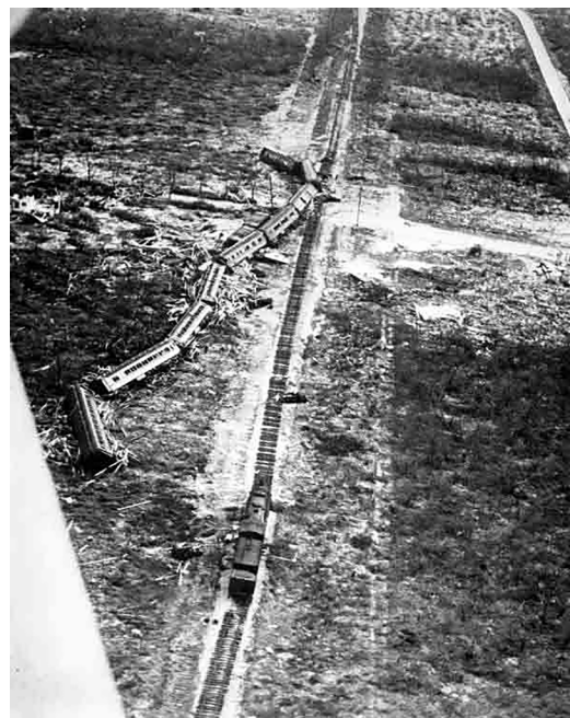
Florida East Coast Railway Overseas Railroad relief train derailed near Islamorada, Florida, during the 1935 Labor Day hurricane.
