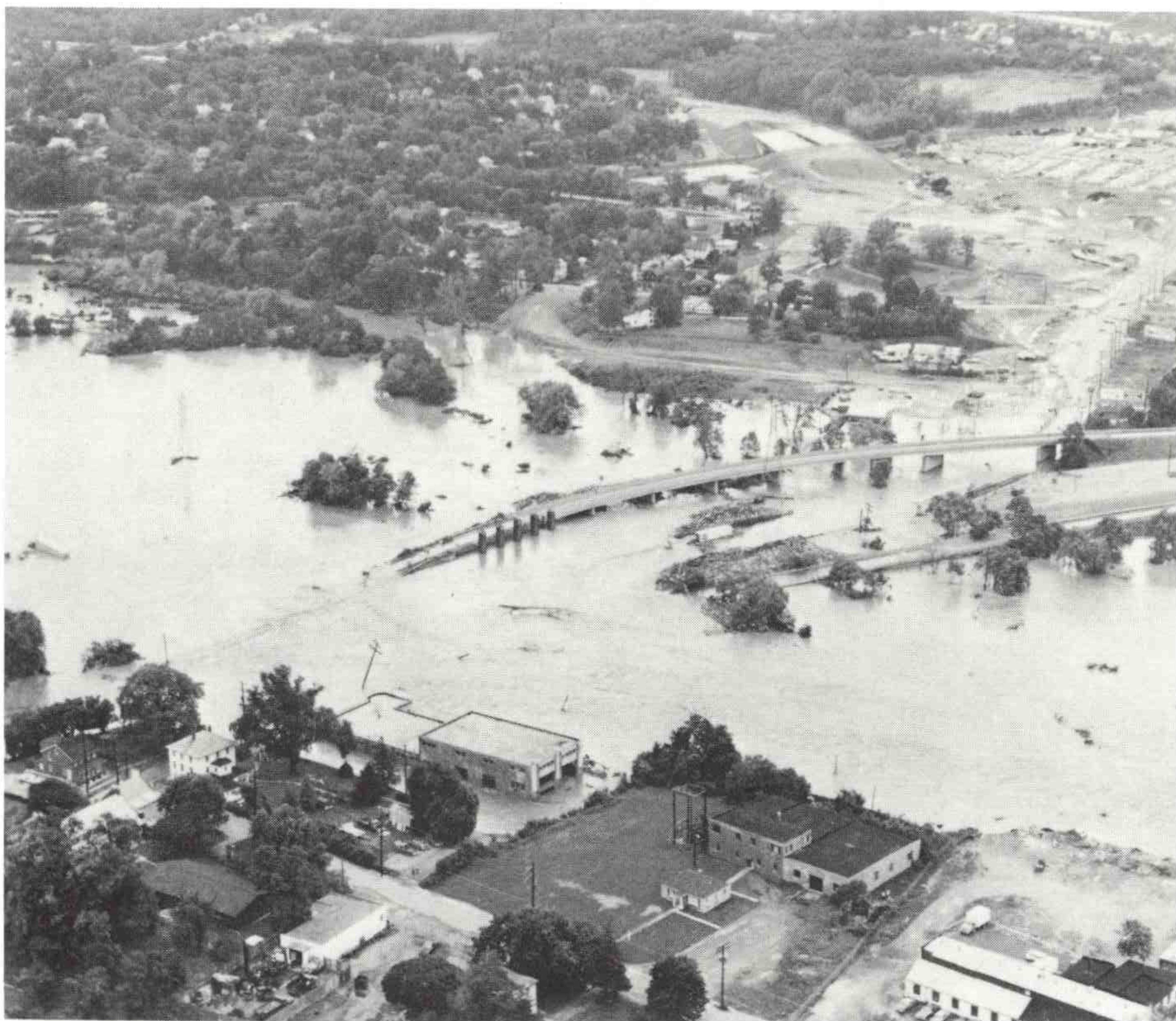
Flood Damage from Tropical Storm Agnes, U.S. Route 1 at Elkridge, Maryland (Patapsco River).
