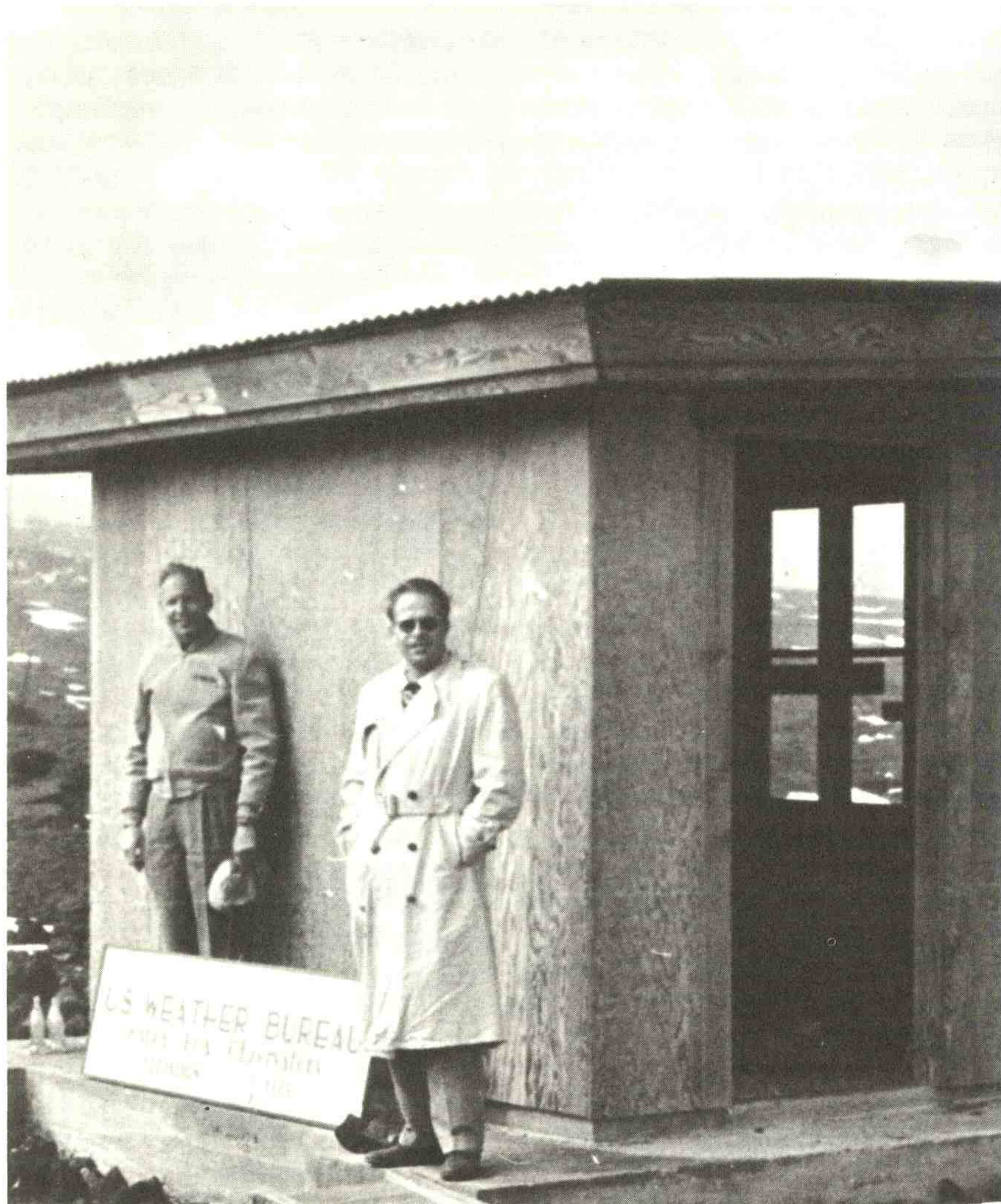
The Mauna Loa summit observatory structure prior to its opening at the 13,453-ft level. R. H. Simpson (left) and Joachim Kuettnner (right).
