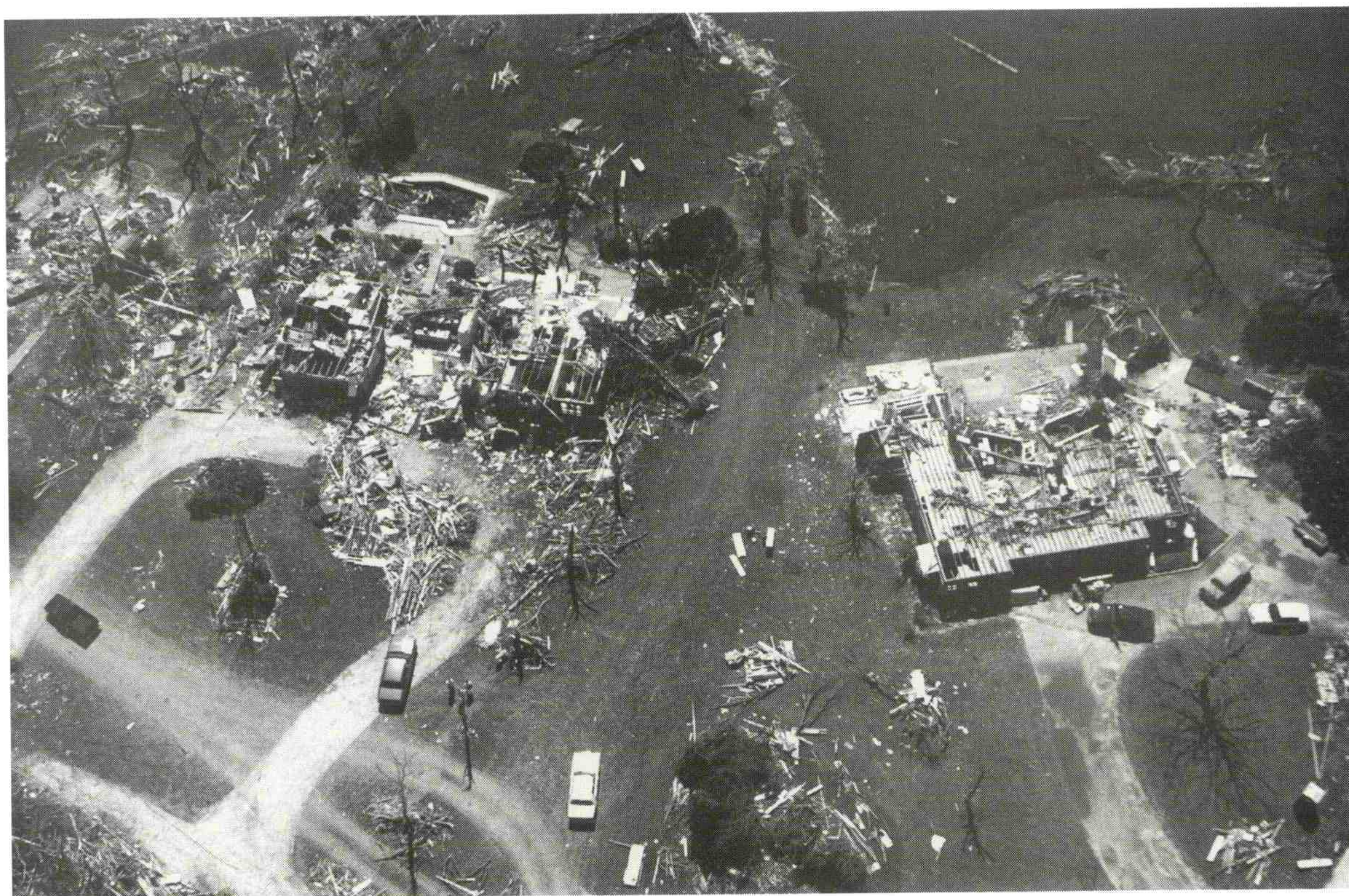
Aerial photograph of damaged homes in the Springdale Subdivision southwest of Andover. Photograph courtesy of Brian Smith, NSSFC.
