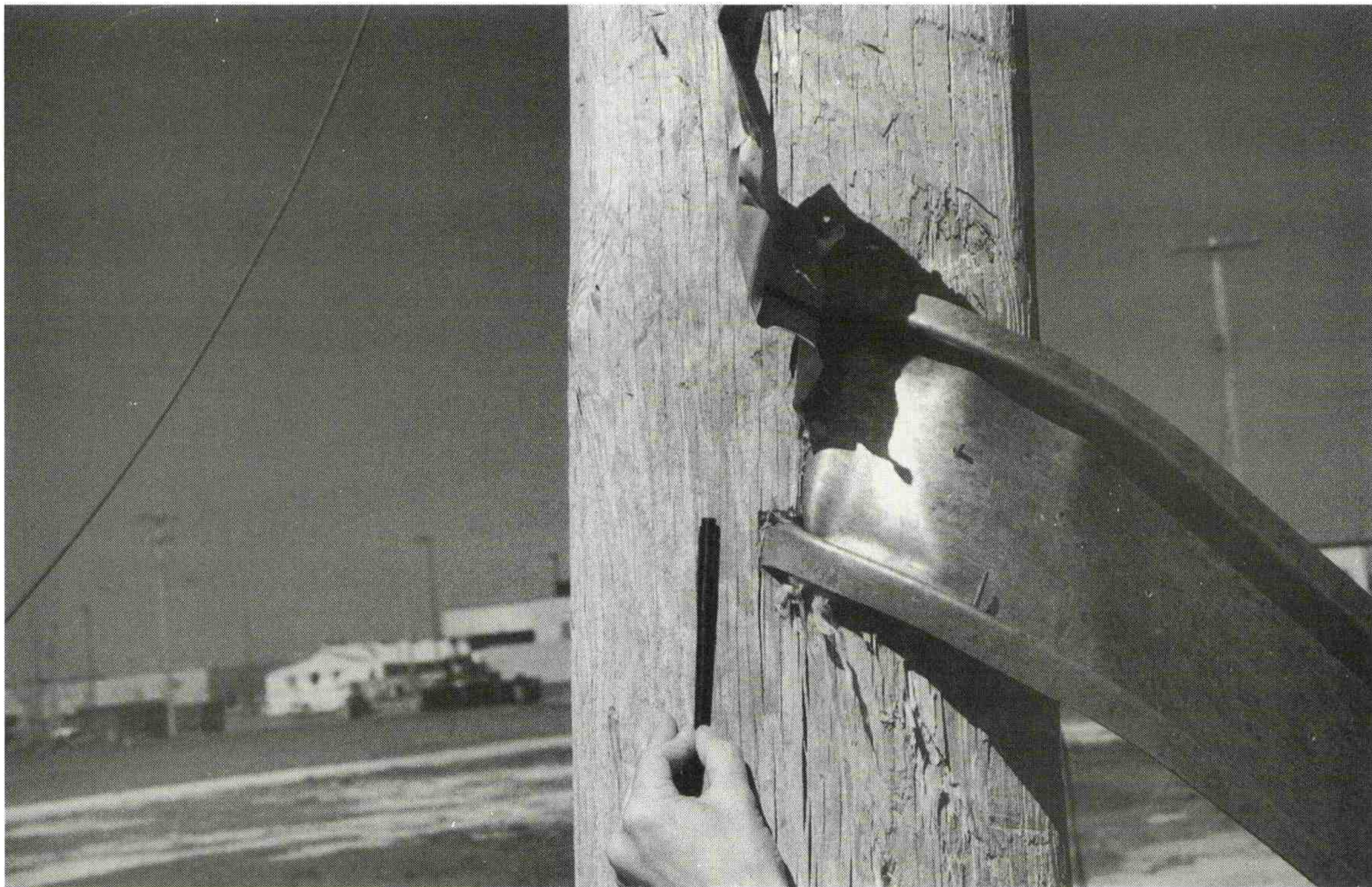
Large metal projectile imbedded in a telephone pole (McConnell Air Force Base). Photograph courtesy of John Sokich, NWS.
