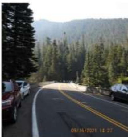
Photo 5. Road conditions along the top surface of the bridge
