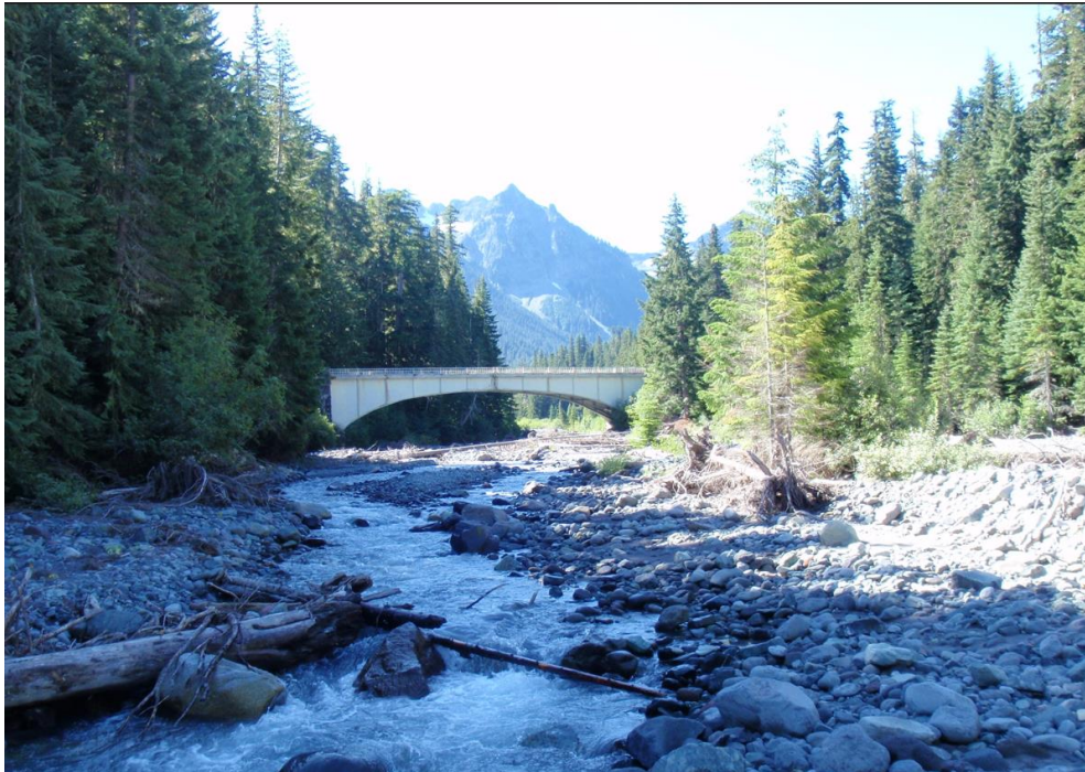
Figure 2. Frying pan Creek bridge and surrounding habitat as viewed looking upstream.
