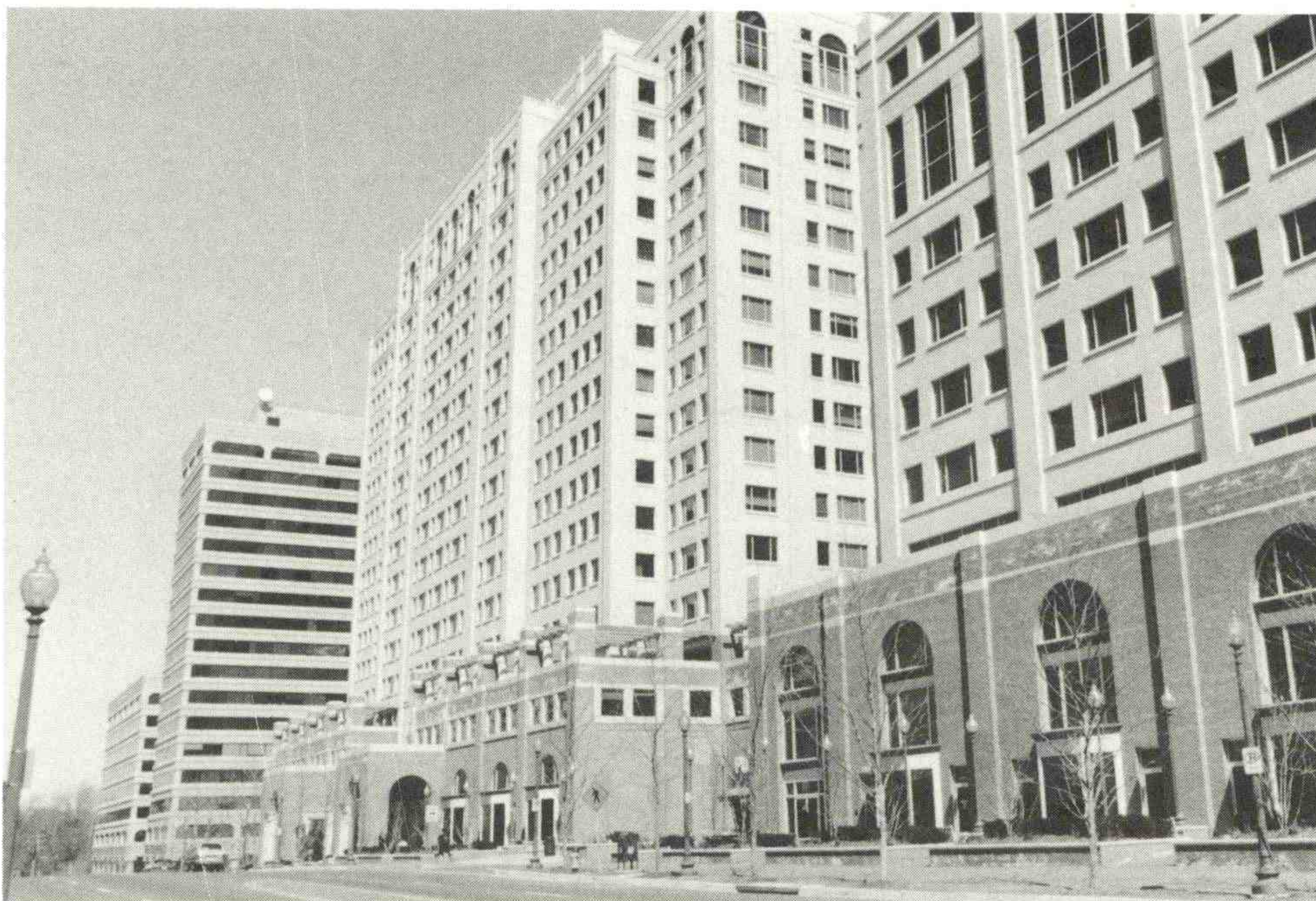
ARL's Headquarters Division is now located in the NOAA Silver Spring Metro Center Building 3.
