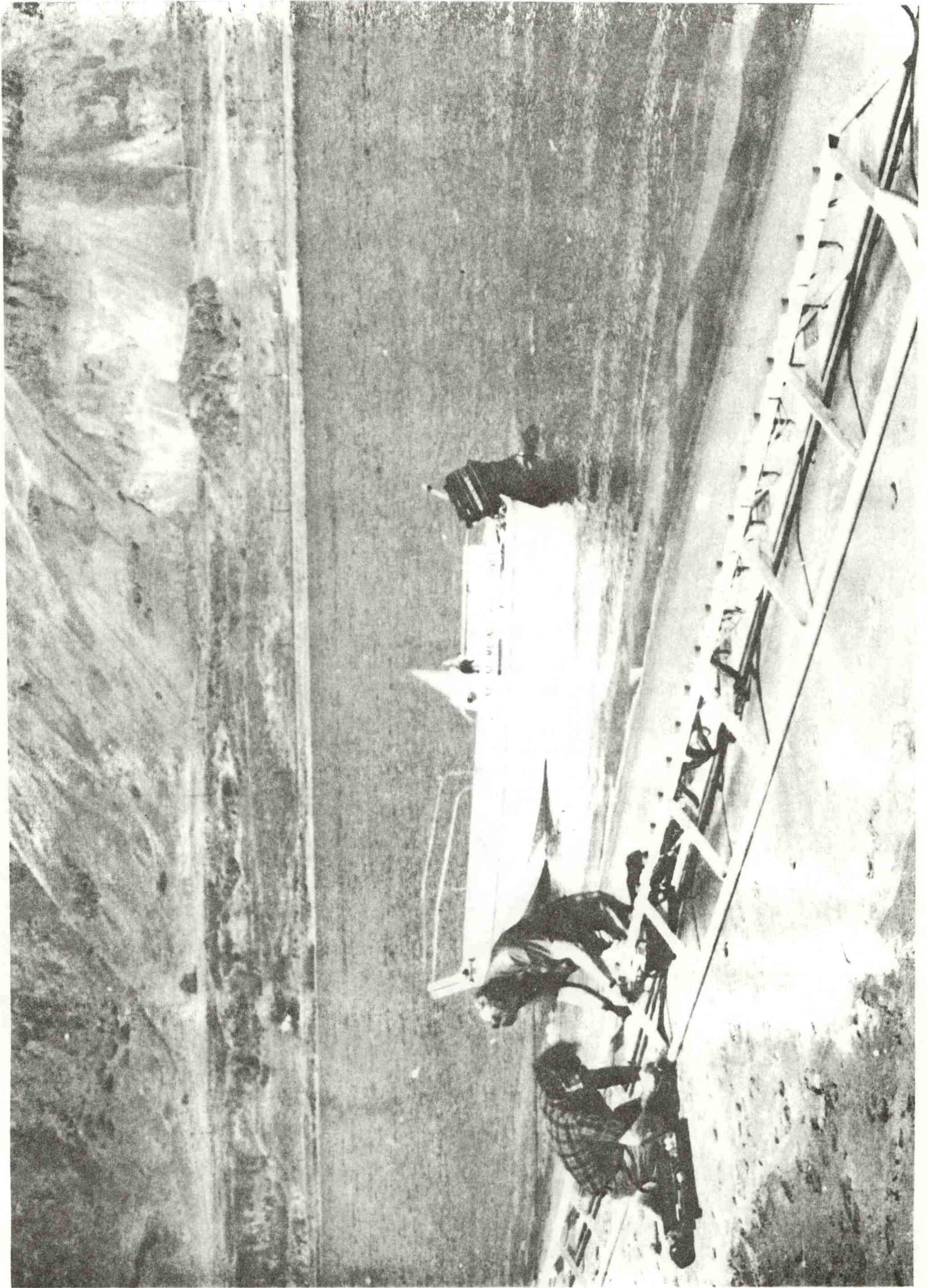
Figure 4.--Twenty-transducer sonic array used near shore 2 km upstream from The Dalles Dam, 1985; Benmar DR-680 with sequencing transducers (from Marshall 1976).
