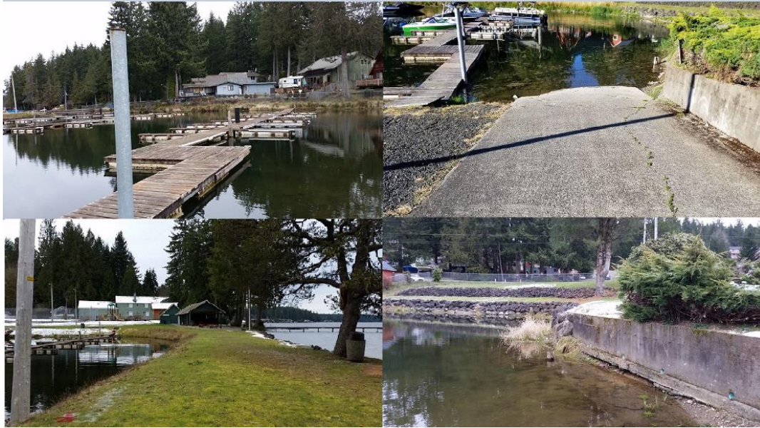
Figure 4. Site photos at Paradise Estates Marina from the ground showing existing ramp, floats, piles, and retaining wall.
