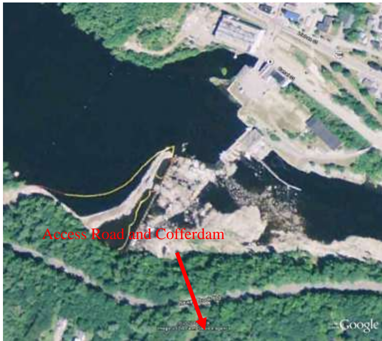
Figure 1. Aerial photo depicting the footprint of the project to rehabilitate the timber crib spillway at the Worumbo Project. The date that this image was taken (8/31/11) is the day after Tropical Storm Irene moved through the area.
