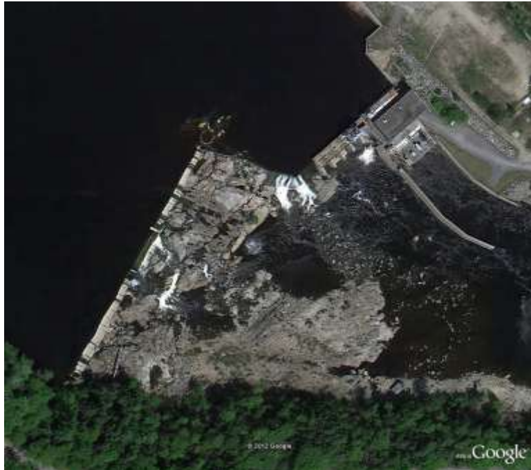
Figure 2. An aerial image of the completed concrete spillway at the Worumbo Project in May of 2012.
