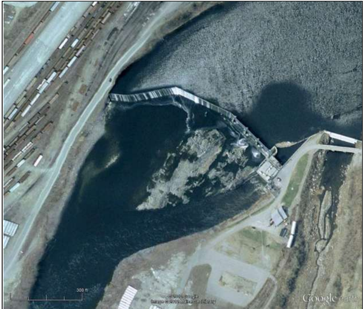
Figure 2. Photograph of Hydro-Kennebec Project.
