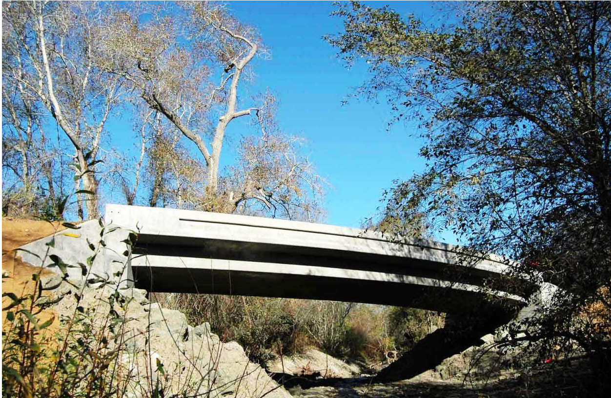
Figure 9. This vehicular bridge over Santa Rosa Creek on Ferrasci Road replaced an at-grade, culverted road crossing that impeded fish passage. Santa Rosa Creek is a Core 1 watershed within the San Luis Obispo Terrace BPG. Photo: Bobby Jo Close, San Luis Obispo County.
