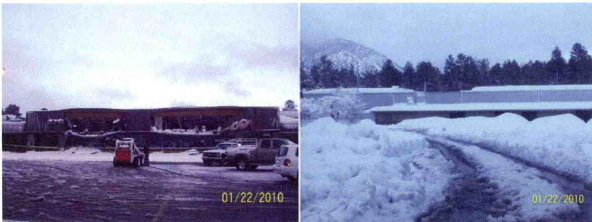
Fig. 24. Roofs of several business in Flagstaff collapsed, including a fabric and bookstore (left), and a community ice rink (right).
