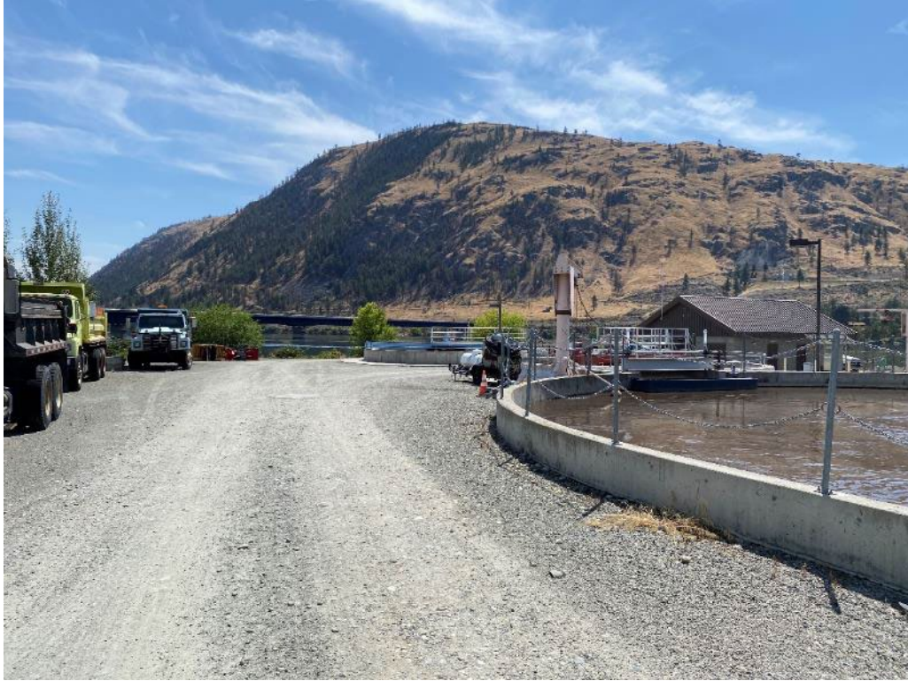
Photograph 1: Southeast view of WWTP
