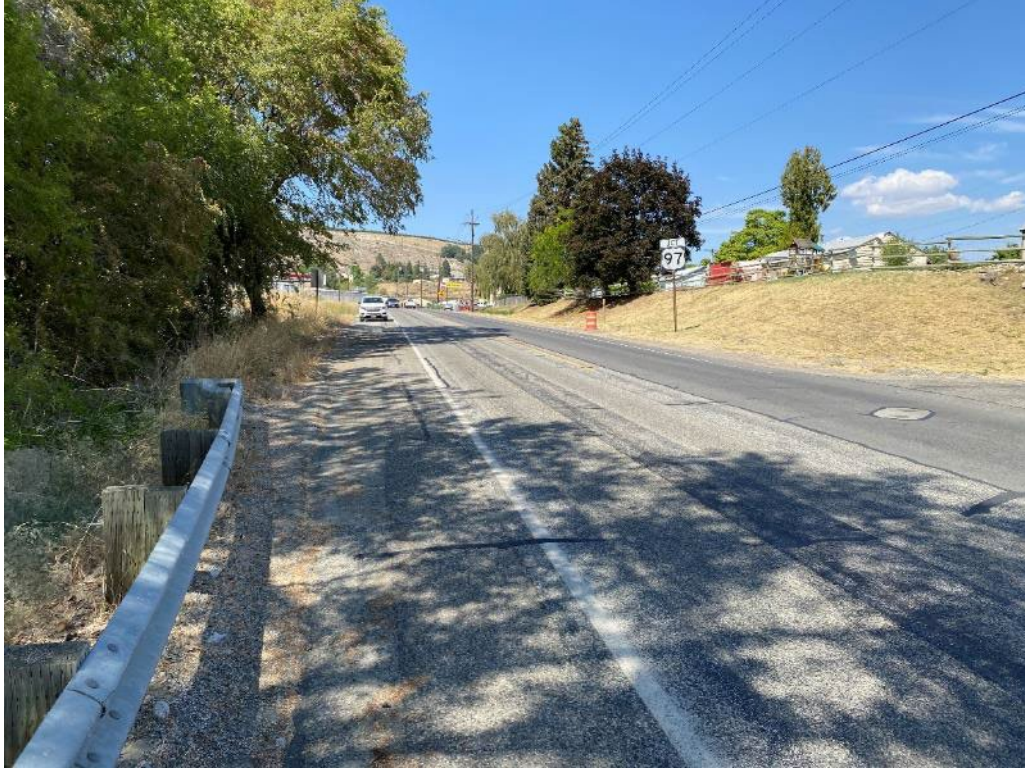
Photograph 5: North view along Bridge Street over Swamp Creek
