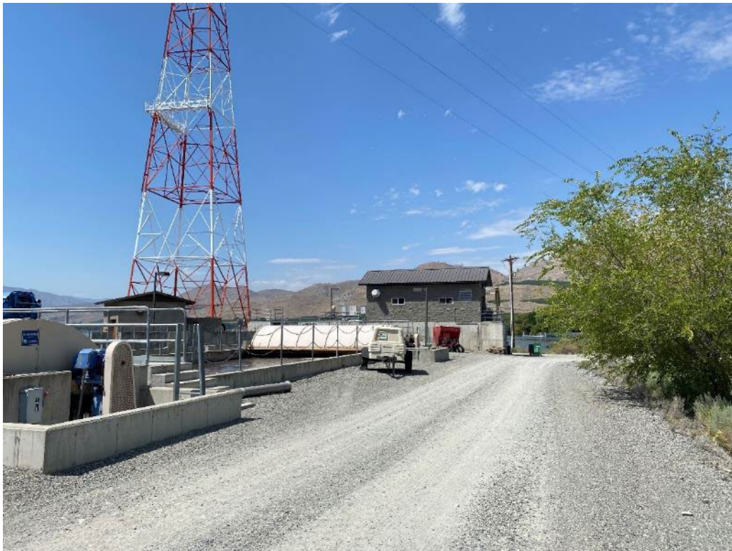
Photograph 2: Northwest view of WWTP showing communications tower
