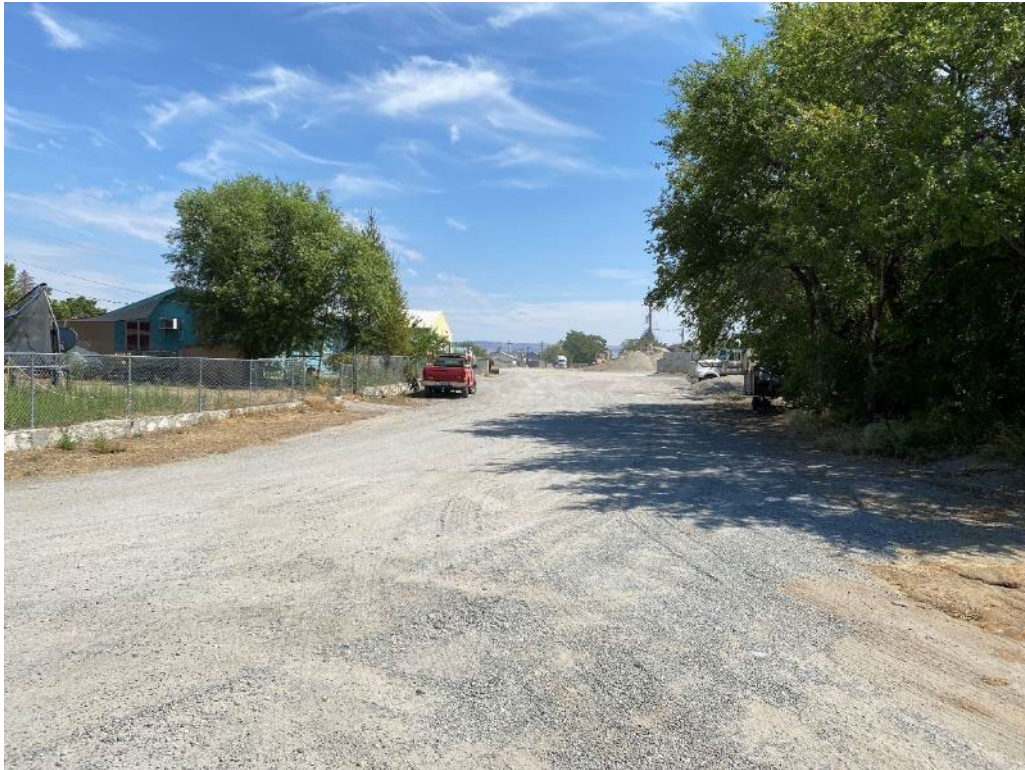
Photograph 4: Ansel Avenue W, road leading to WWTP entrance road
