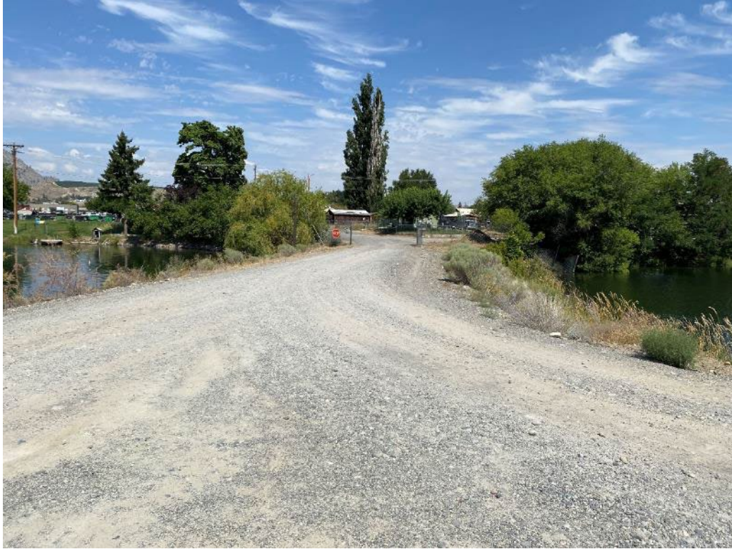
Photograph 3: Northeast view of entrance road to WWTP
