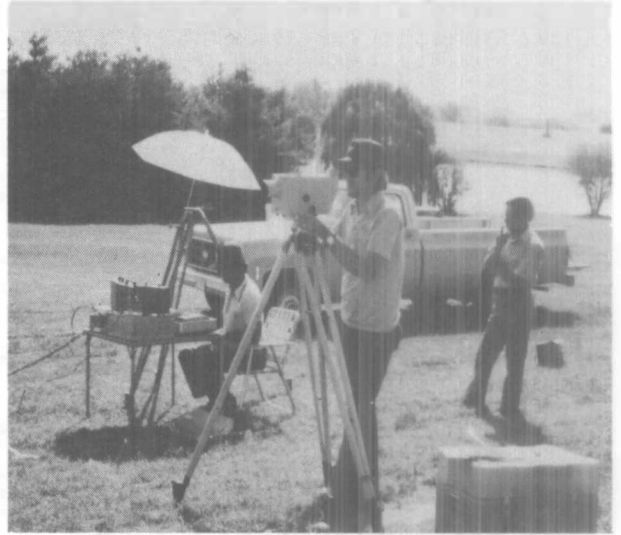
Figure 4.—Leveling team in operation.
