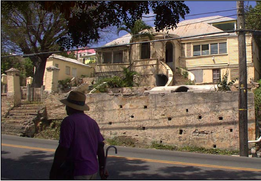
Figure 28: Many houses are still abandoned and damaged due to Hurricane Hugo.
