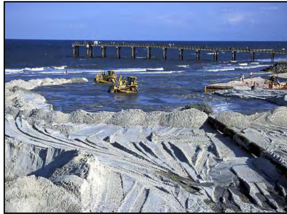
Figure 9: Sand dike construction.
