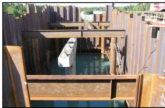
Internally Supported Cofferdam. Source: www.kenairriverbridge.com
