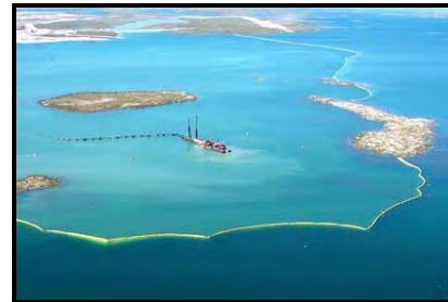
Use of a turbidity barrier for a large-scale project. Source: http://www.geomembranes.com/images/path_product/Ocean1-3.jpg
