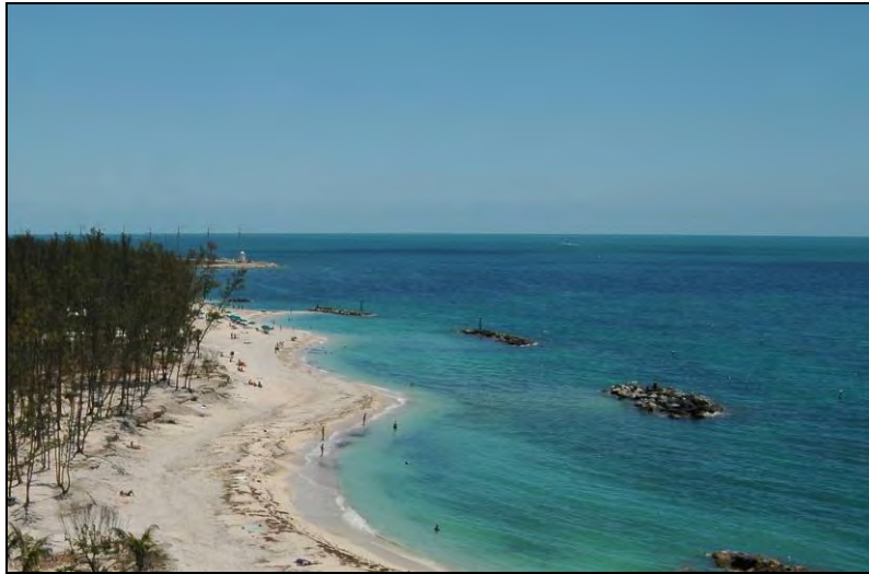
Figure 13: Sub-aerial breakwaters, Key West. Source: PBS&J
