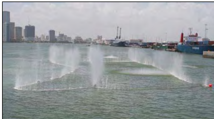
Figure 6: Blasting in Miami Harbor. Source: USACE
