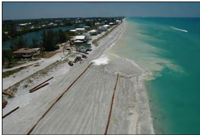
Figure 7: Beach Nourishment Project. Source: PBS&J
