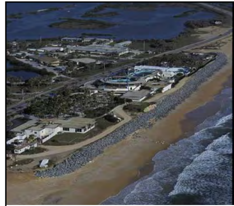
Figure 11: Revetment at Marineland. Source: PBS&J
