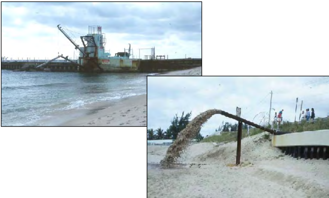
Figure 5: South Lake Worth Inlet Sand Transfer Plant (above left) and discharge pipe (above right). Source: Palm Beach County
