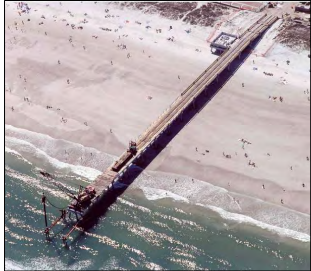
Figure 14: Pier under construction. Source: PBS&J
