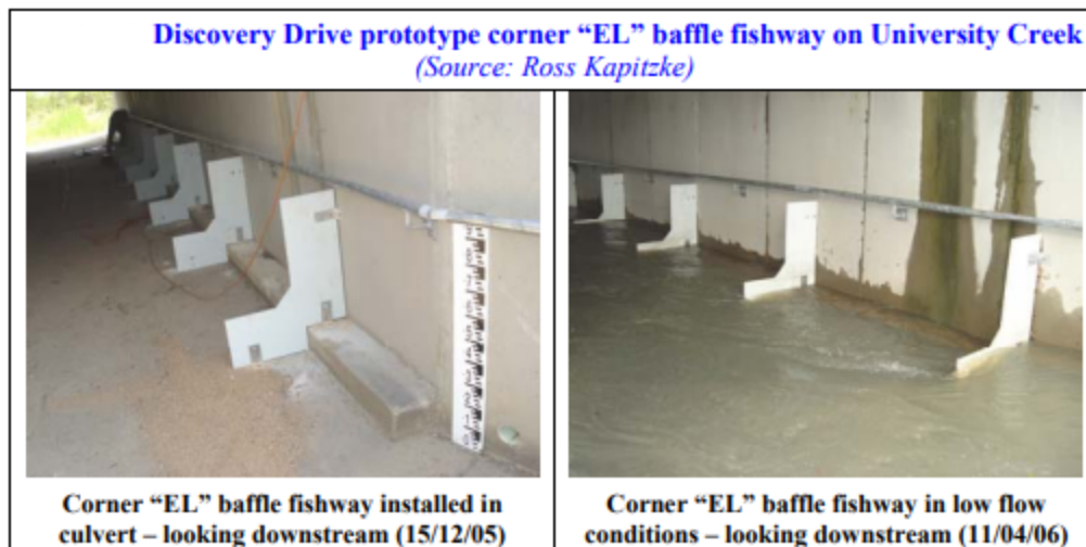
Figure 2. Example of an "EL" style baffle in a fishway
