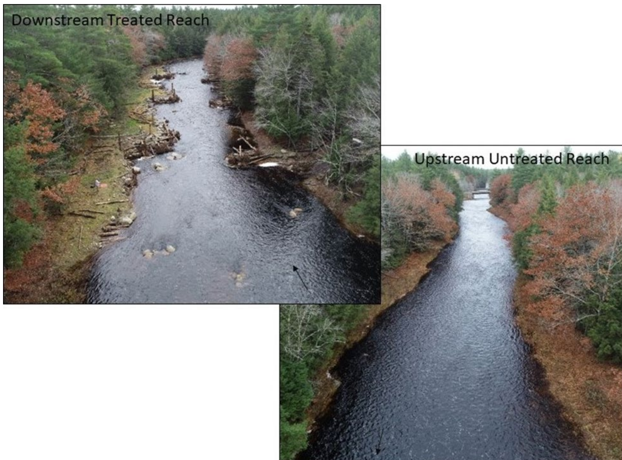
Figure 3.3.3. Drone's eye view of the Narraguagus River Restoration Project at Rt 9 Pilot site showing the engineered log jams in the left photo and the untreated reach immediately upstream of the treatment site.
