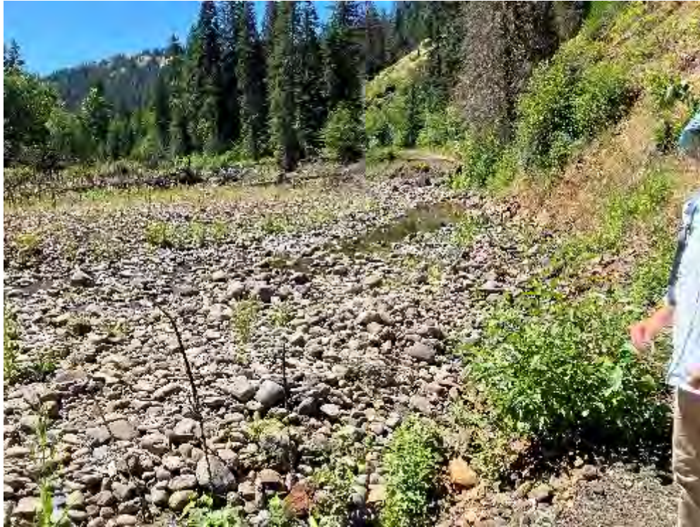
Figure 1-8: Road washout at MP 2.02, looking upstream. The main river channel is currently well to the east (left on this photo).
