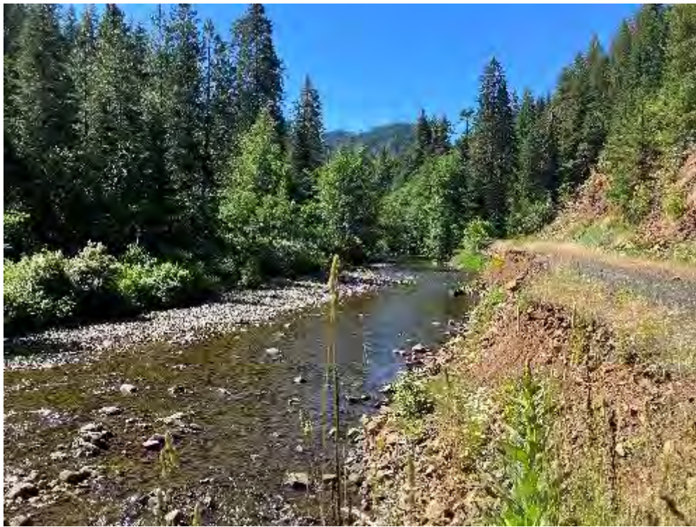
Figure 1-42: Road and bank erosion at MP 3.23
