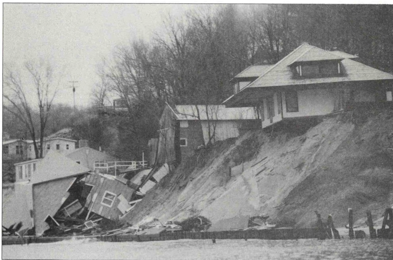
Figure 20. Flooding due to a storm surge in western Lake Erie during high lake levels in 1979 (top). Erosion and damage on the eastern shore of Lake Michigan caused by the combination of record high water levels and winter storms during late 1985 (bottom).
