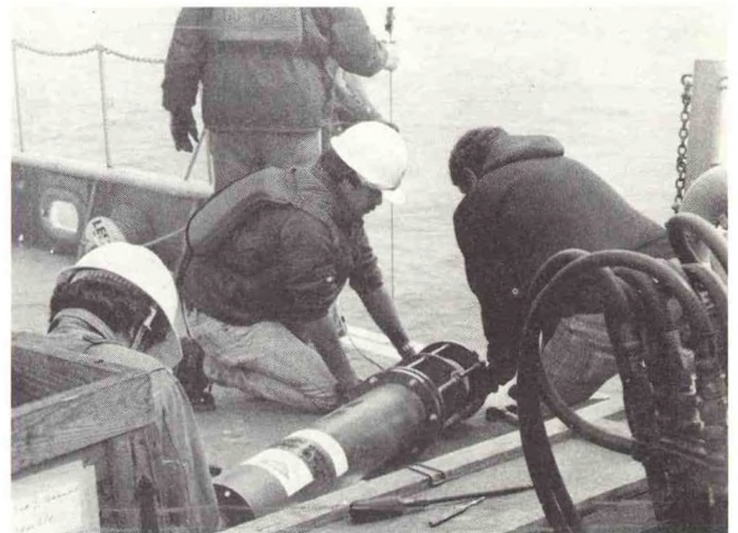
Deployment of a current meter in Lake Michigan. These meters record currents and temperatures for 1 year and provide the fixed array data used in water movement studies.
