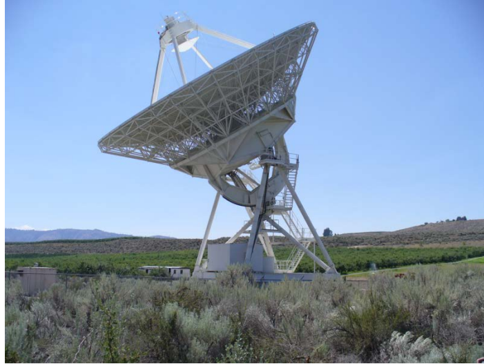
Figure 4 - 7614 VLBA, view looking to the south.
