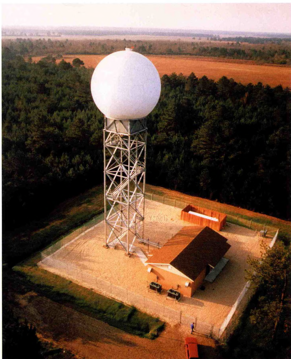
Figure 3-DOT-2. FAA Terminal Doppler Weather Radars provide supplementary wind and precipitation conditions for airport approach and departure.
