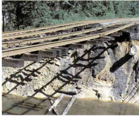
Figure 3-DOT-6. Track trussel washed out by flood waters.
