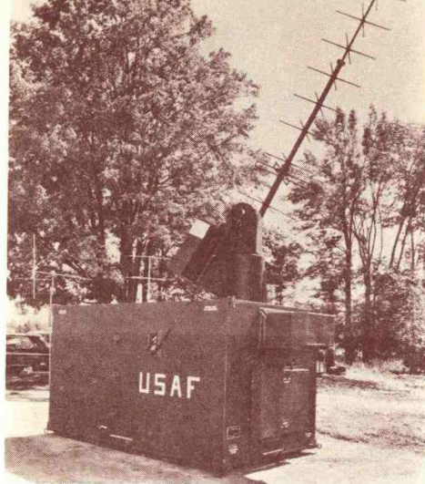
Spiral antenna atop of APT van picks up signals from weather satellites.
