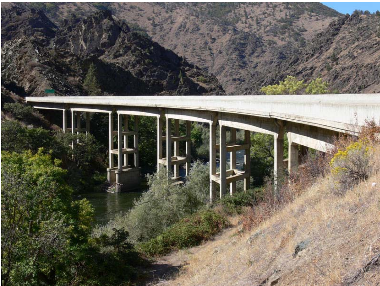
Figure 2. Existing SR 263 bridge over the Klamath River (Caltrans 2016).
