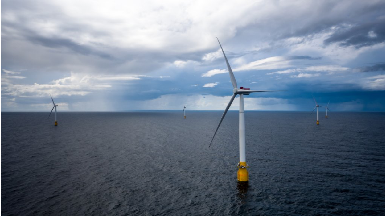
Figure 3: Hywind Scotland (Floating Offshore Wind Energy: A Policy Blueprint for Europe, 2016).
