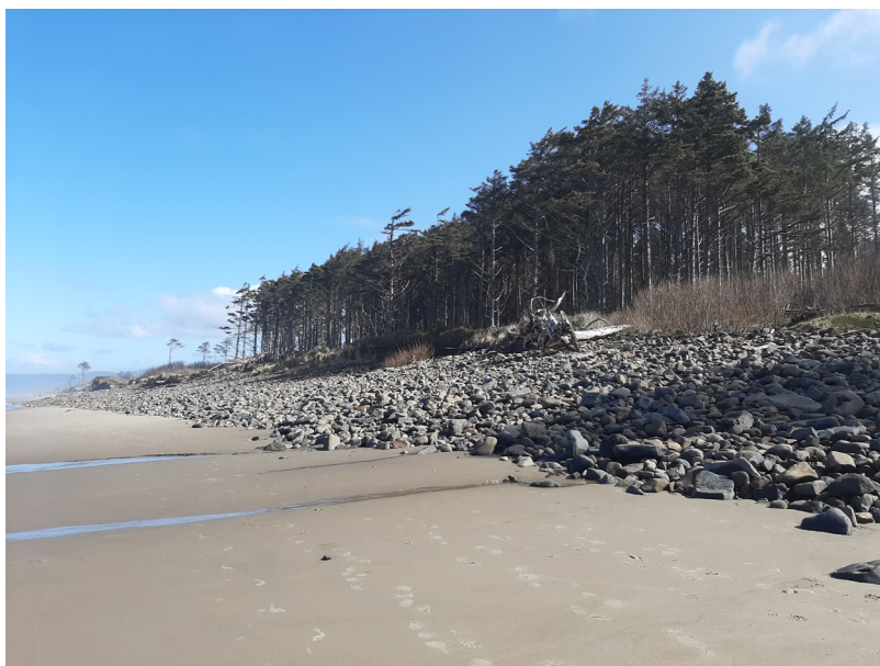
Figure 5. Dynamic revetment at Cape Lookout State Park, Tillamook County, Oregon, March 2021. Photograph by Hailey Bond.
