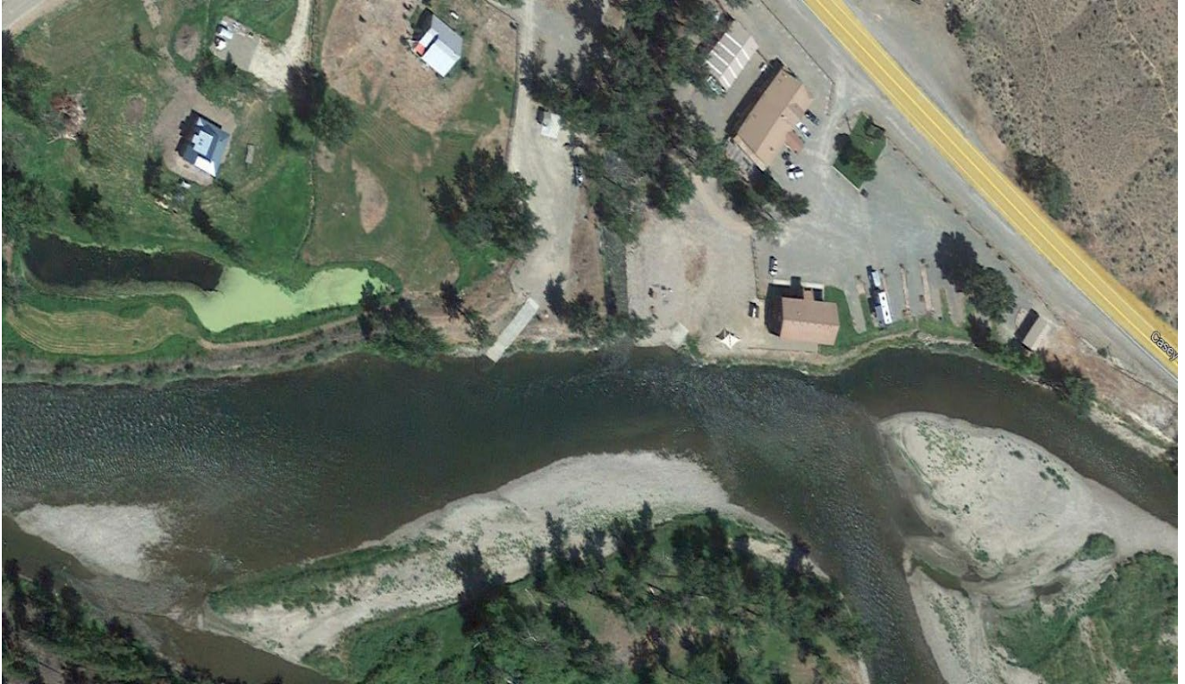
Figure 2. The IDFG North Fork boat ramp on the Salmon River just downstream of the confluence of the North Fork Salmon River. The yellow roadway is U.S. Highway 93 North (Google Earth July 2016).
