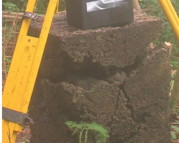
Figure 5. Condition of SARIGAN AZIMUTH mark.
