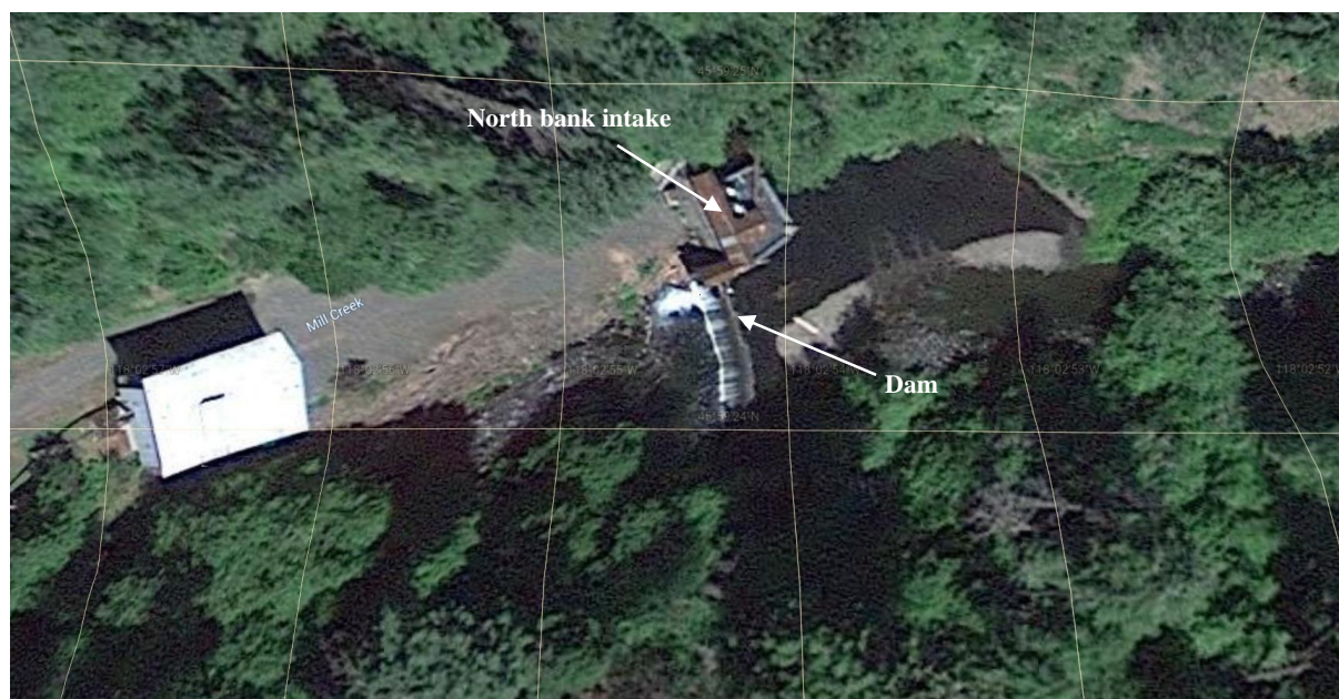
Figure 3. Aerial photo of site, showing dam and intake on north bank of Mill Creek. Gravel bars evident upstream.
