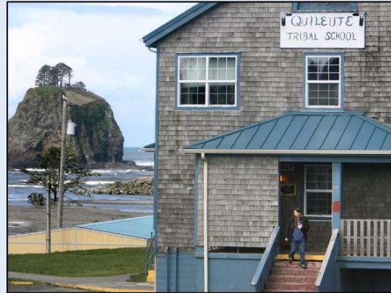
Figure 13. The Quileute Tribe is currently working to relocate their Tribal School out of the tsunami hazard area, as part of the Move To Higher Ground project. Image provided by Tony Overman/ The Olympian , 2021.
