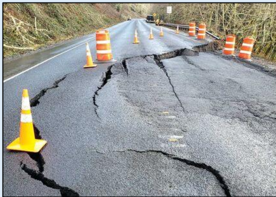
Figure 14. WSDOT works to address a landslide on State Route 401, along the shoreline of the Columbia River estuary. Image provided by the Wahkiakum County Eagle , 2021.
