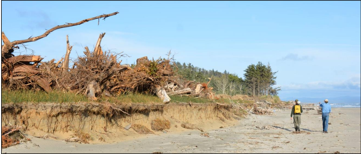
Figure 23. Erosion is a chronic issue across Washington's Pacific Coast. The COHORT would help communities access funding and develop long-term, multi-benefit solutions for hazards problems such as these. Image provided by the Washington State Department of Ecology's Coastal Monitoring & Analysis Program, 2018.
