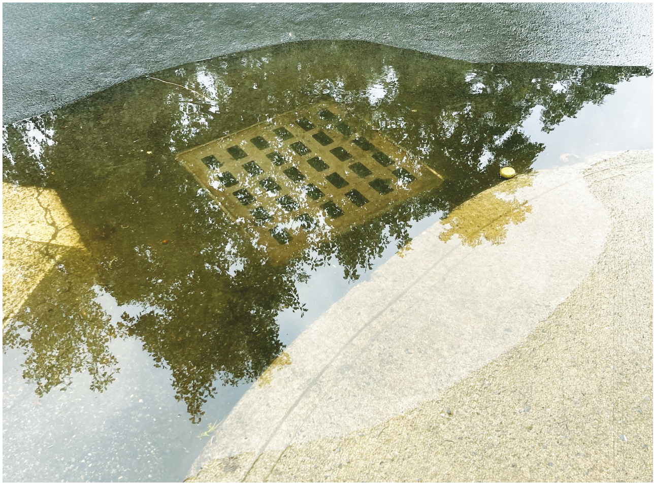
Storm drain back up due to an extreme high tide. Image credit: Jessica Kuonen, New York Sea Grant.
