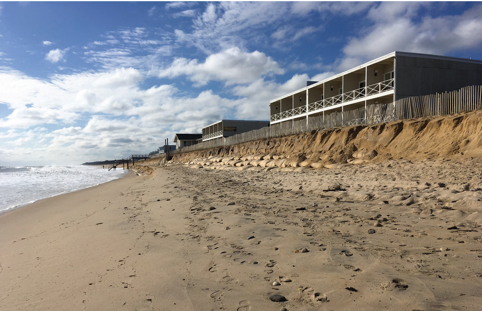
Exposed sand bags due to beach erosion. Image credit: Kathleen Fallon, New York Sea Grant.
