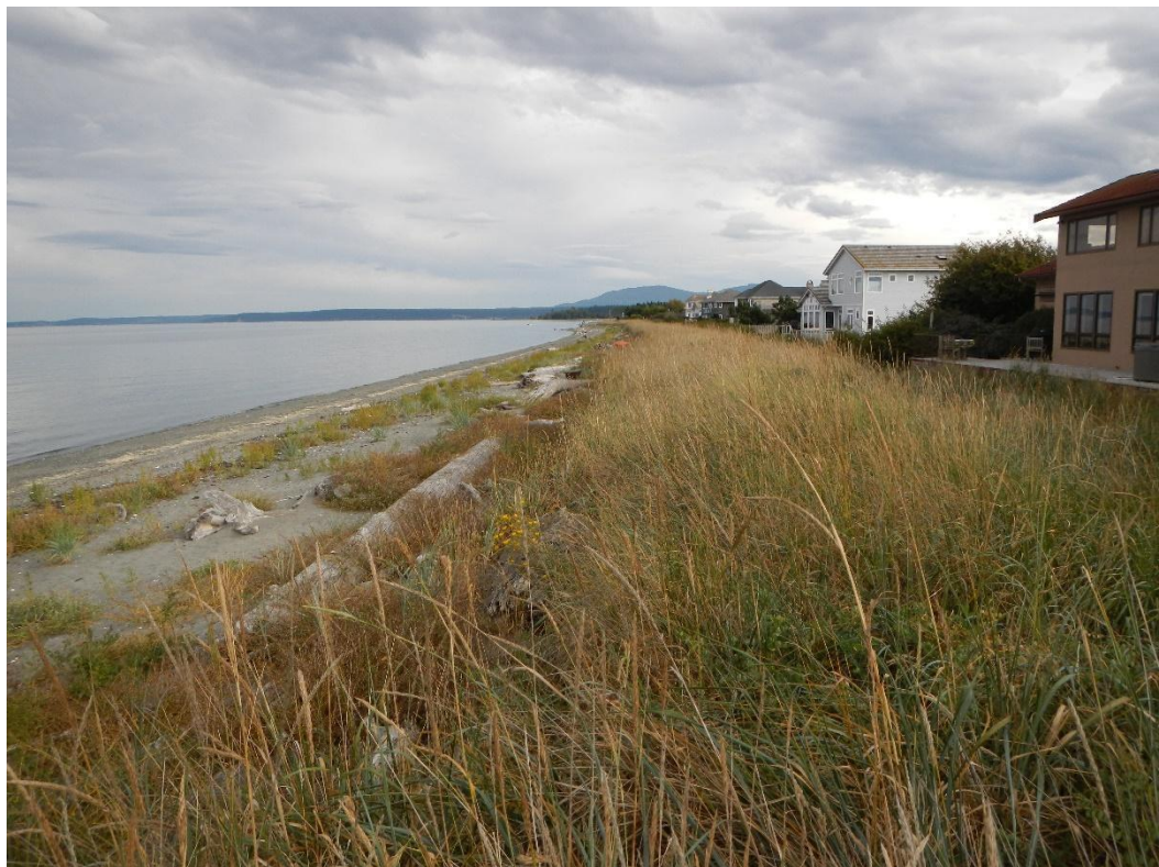
Figure 8. A soft shore engineered berm protects 15 parcels along a stretch of shoreline near Sequim, Washington. This project requires collaboration and coordination between neighbors to fund, build and maintain the berm, providing a template for coordinated approaches that may be required as sea level rises. August 2013 photo by Ian Miller, Washington Sea Grant.
