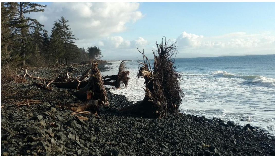
Figure 9. A cobble "dynamic revetment", with placed large wood, built along the shoreline near North Cove, Washington and designed to reduce erosion. Photo by Jackson Blalock, Washington Sea Grant.
