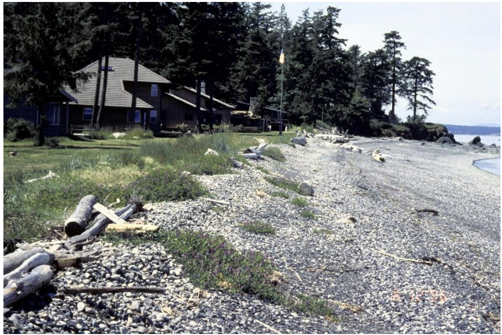
Figure 11. A cobble berm installed in 1992 at a site on the north side of Orcas Island, Washington replaced shoreline armor. This soft shore project has performed well since installation, providing erosion control and flood risk reduction at this site (Johannessen et al., 2014). 2006 photo by Hugh Shipman, Washington Department of Ecology.
