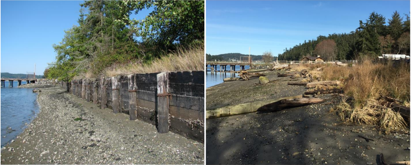
Figure 10. Before (left panel) and after (right panel) the removal of shoreline armor and implementation of soft shore techniques at Cornet Bay near Deception Pass on Whidbey Island. The presence of large wood, beach wrack and vegetation on the upper beach suggests removing the shoreline armor improved ecological function along this stretch of shoreline. August 24, 2009 (left) and February 23, 2016 (right) photos by Hugh Shipman, Washington Department of Ecology.
