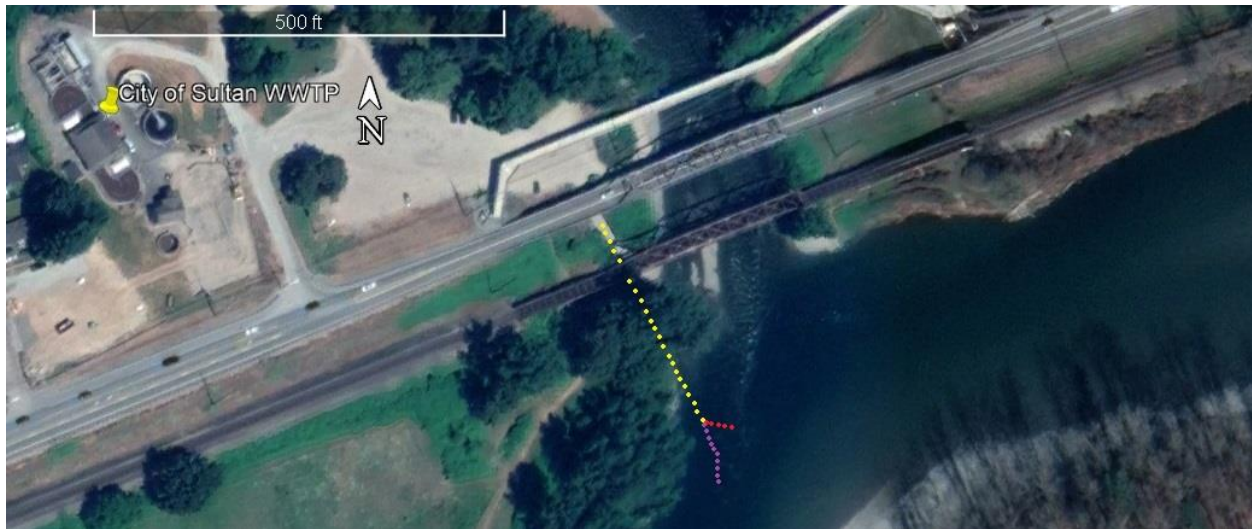
Figure 2. Google Earth photograph showing the City of Sultan’s WWTP, and the approximate positions of the existing and proposed outfall pipes. The yellow dotted line indicates the alignment of the buried pipeline as it crosses the under the bank to its point of connection with the existing (red) and proposed (purple) outfall pipes in the Skykomish River. The Sultan River extends north under the bridges.
