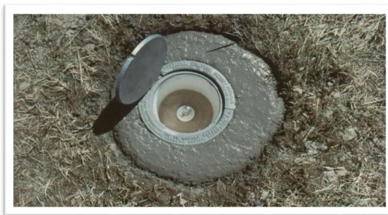
Figure 5-8. Completed deep rod mark, shown with logo cap in open position. Note rod with datum point extending out of greased sleeve; rod assembly is below the soil surface.
