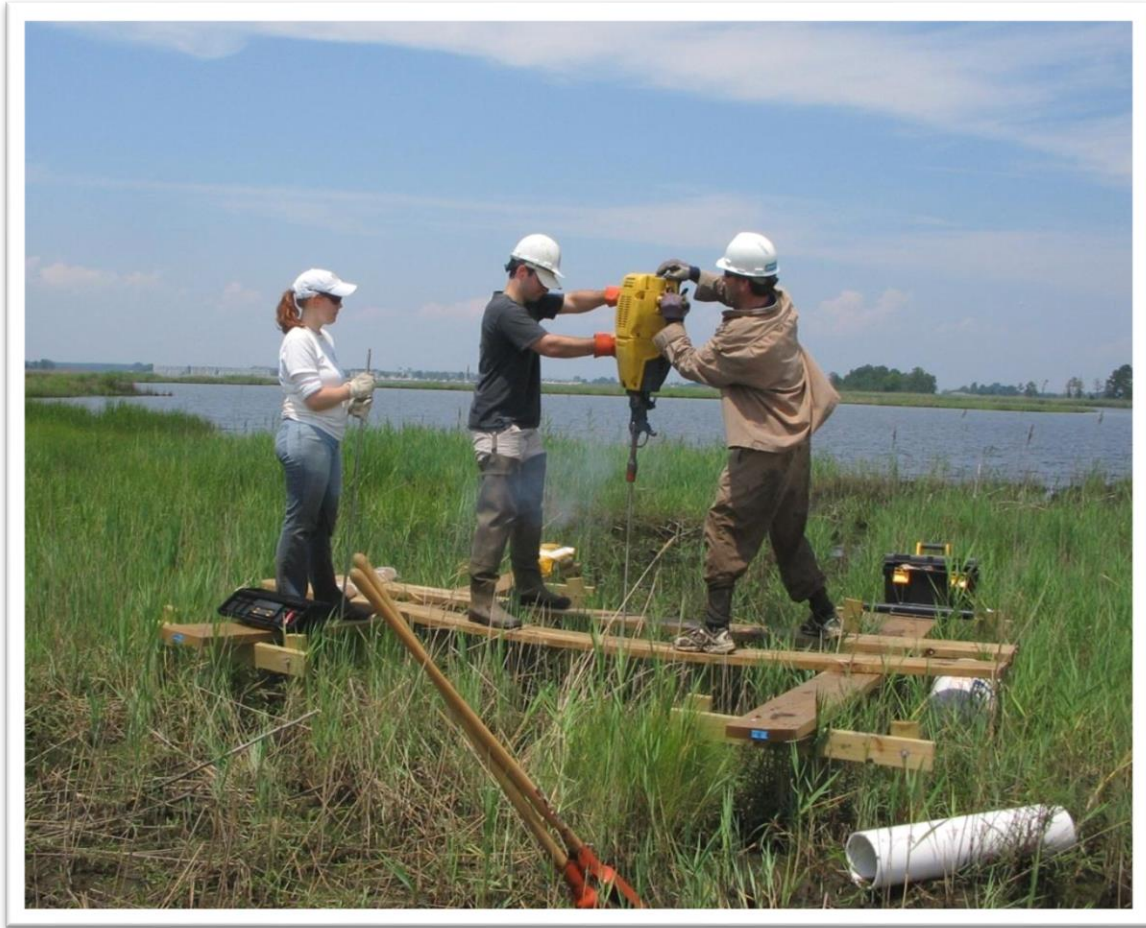
Figure 5-5. Field crew setting a deep rod mark in a Chesapeake Bay wetland, Maryland. Note use of platform to avoid disturbance on wetland soil.
