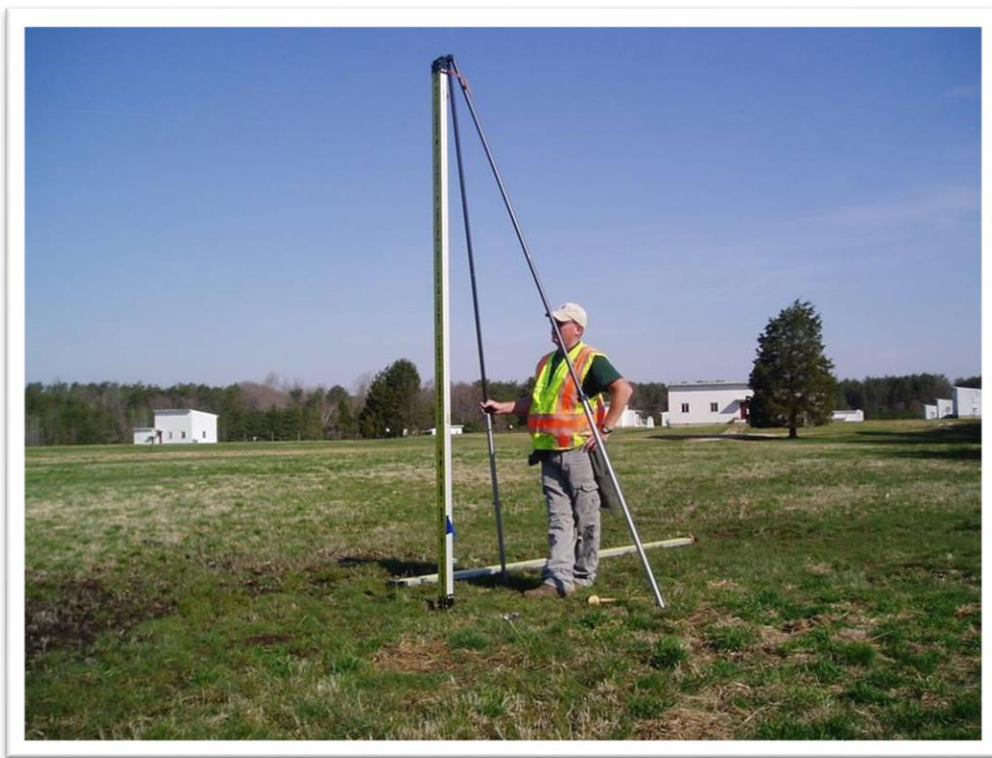
Figure 6-15. Three-meter tall-digital barcode level rod set on turning point, showing brace poles in action. Brace poles ensure immobilization of rod during the leveling operation, keeping the rod plumb.
