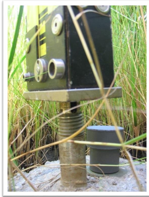
Figure 6-14. Close-up of level rod placed atop a deep rod SET receiver (bench mark). The vertical point of reference is the top-most side of the receiver. The cap to the receiver is shown and has been removed before leveling to the SET.
