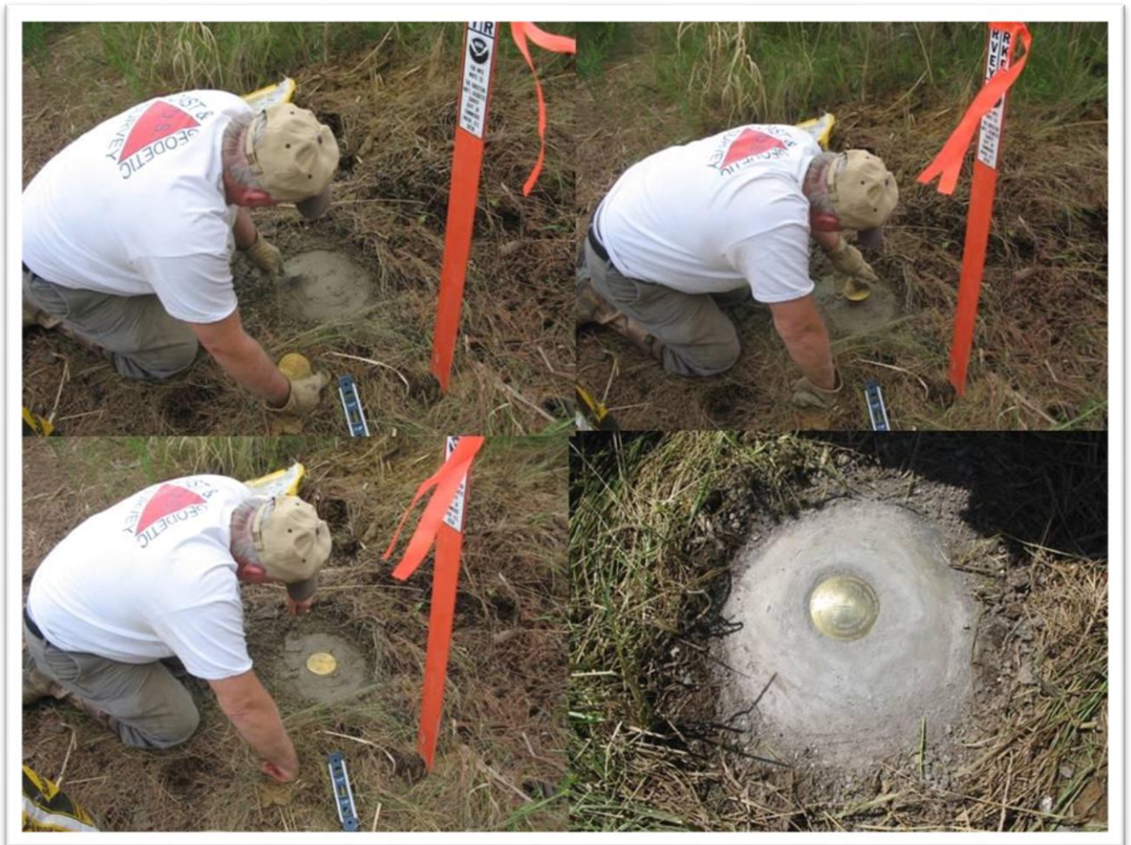
Figure 5-3. Steps involved in finishing the mark: smoothing the top; inserting the marker; final touch-up smoothing the surface; the cured mark. Note witness post to the right of the mark, with flagging.
