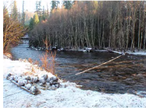
(b) deadman anchor in western Oregon
