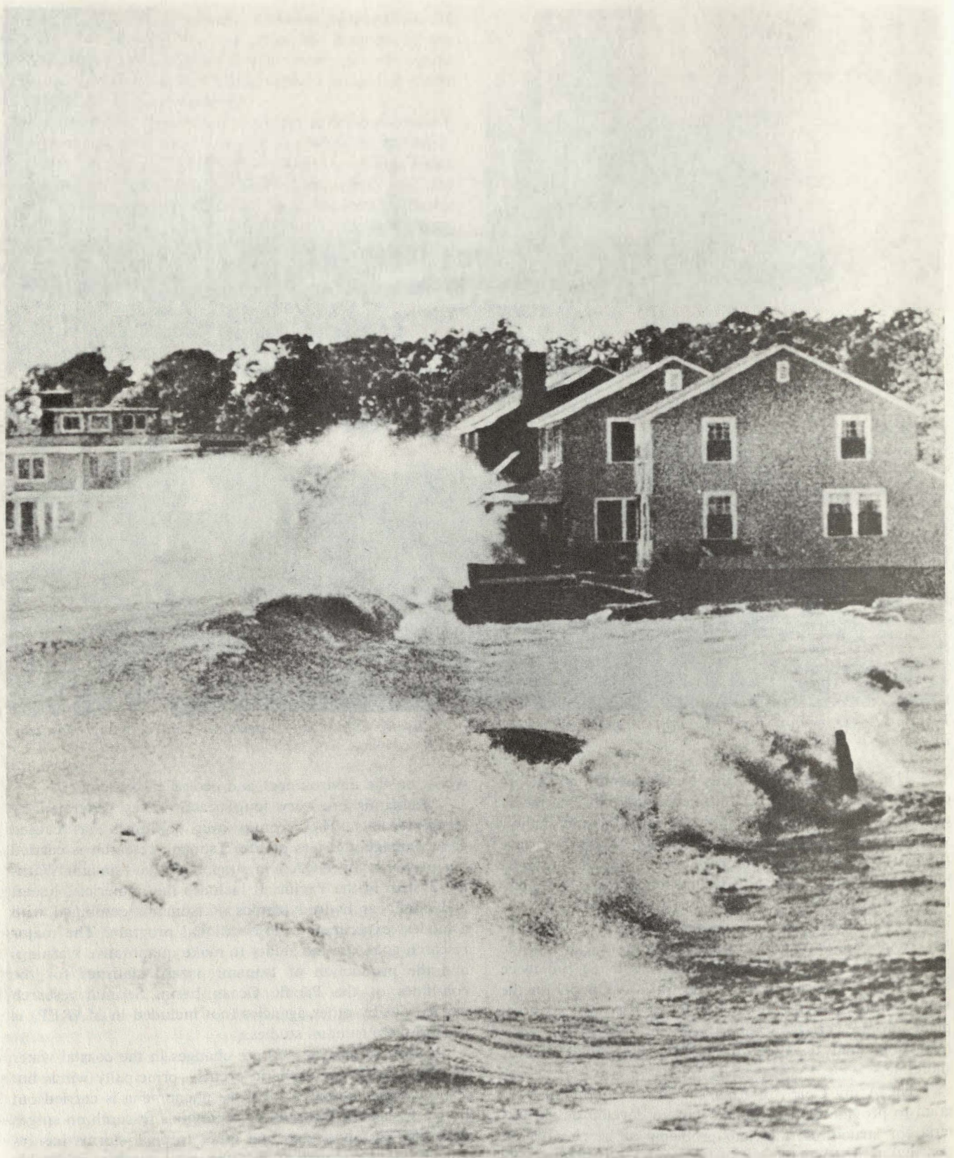
Figure 32.—Hurricane storm surge is the principal mechanism by which low coastal structures are destroyed. Surge associated with a hurricane floods Old Lyme, Conn., on the Long Island Sound north shore.
