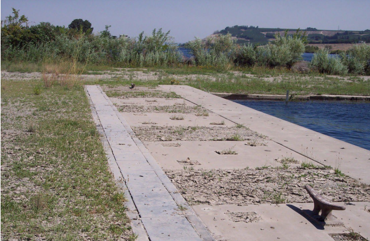
PHOTO 5: Port of Benton Barge Slip and surrounding vegetation/gravel, looking north(7/17/2014)
