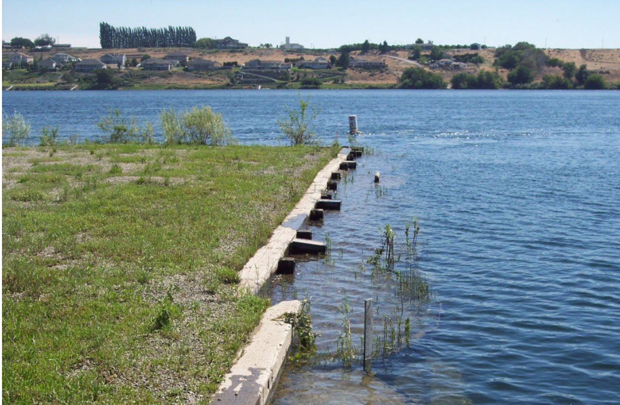
PHOTO 7: Port of Benton Barge Slip with surrounding aquatic vegetation, looking east (7/17/2014)
