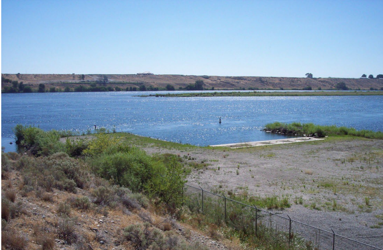
PHOTO 1: Port of Benton Barge Slip looking east-southeast (7/17/2014)
